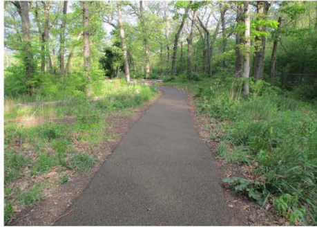
Flexible Porous Surfacing
