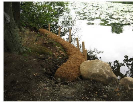
Single Coir Fascine
