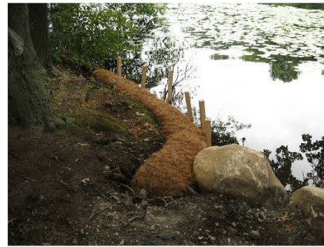
Single Coir Fascine
