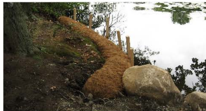
Single Coir Fascine
