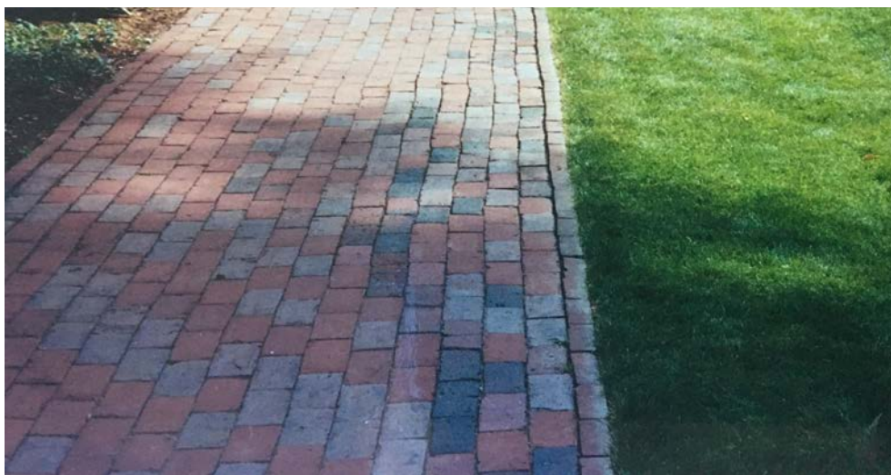
1999 image of brick walkway adjacent to the Whittemore-Robbins House with flush brick edging
