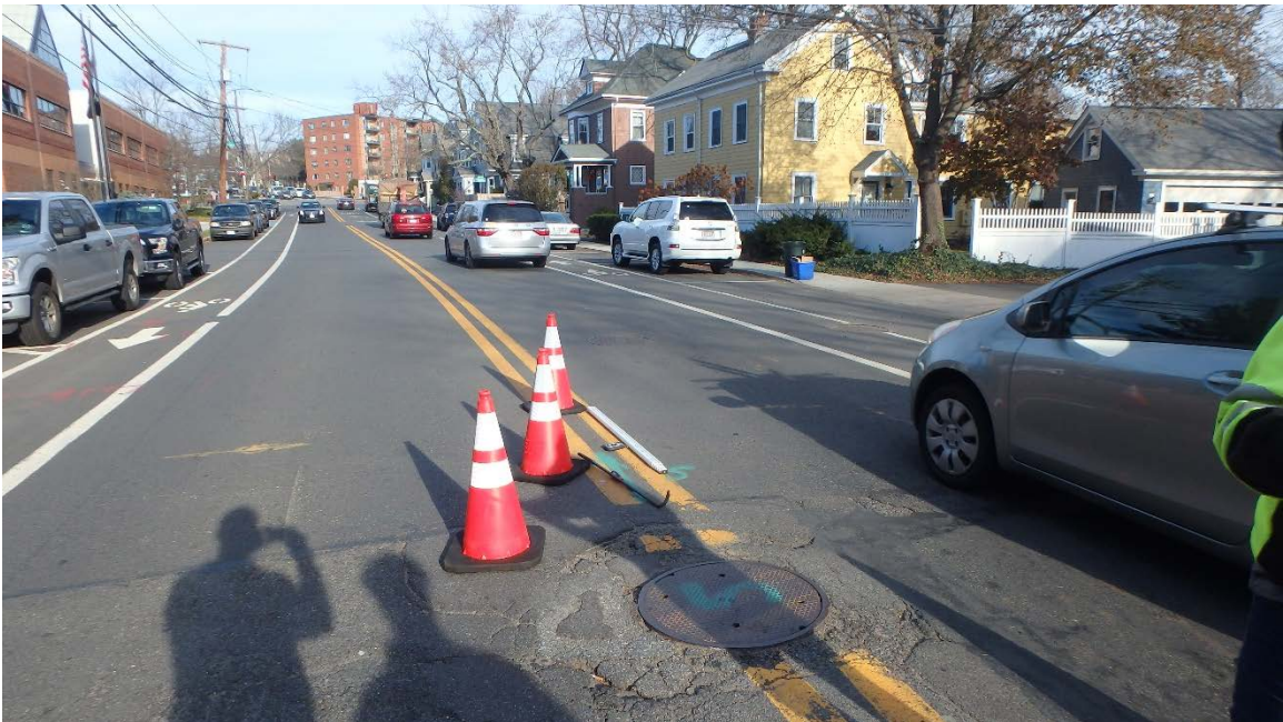
EXISTING MANHOLE MA-121 SHEET C-1 STATION 2+86 AREA PHOTO
