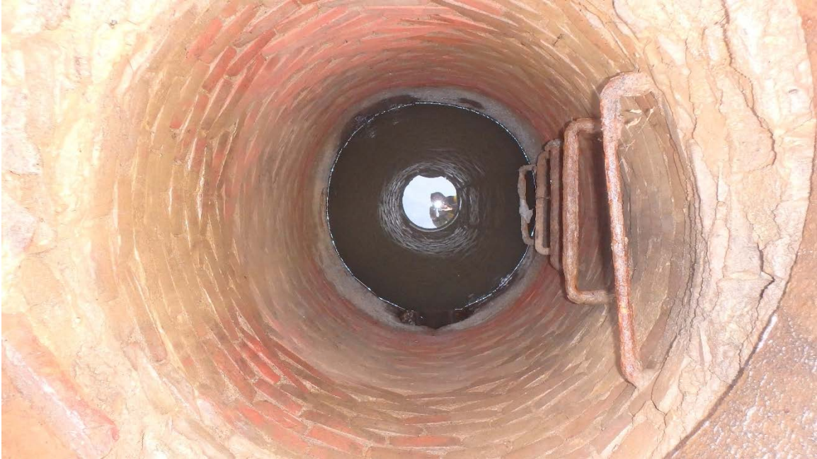
EXISTING MANHOLE MA-120 SHEET C-1 STATION 2+48 INTERNAL PHOTO
