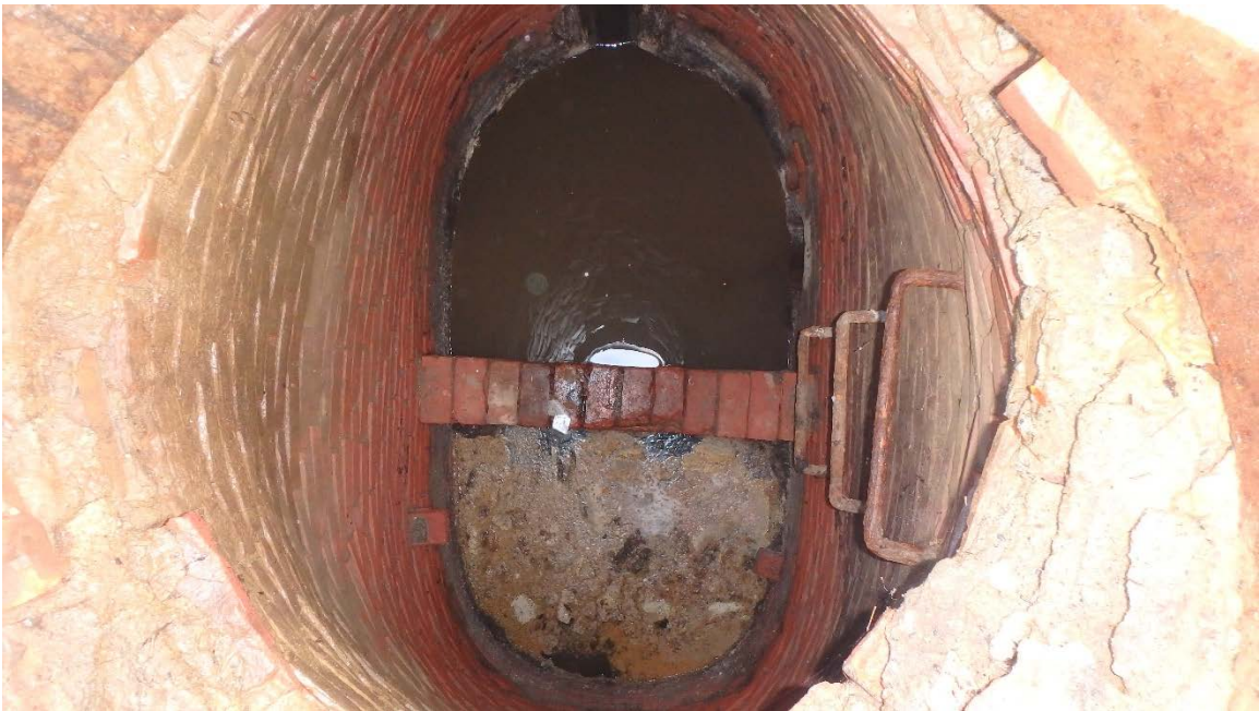
EXISTING MANHOLE MA-121 SHEET C-1 STATION 2+86 INTERNAL PHOTO #1
