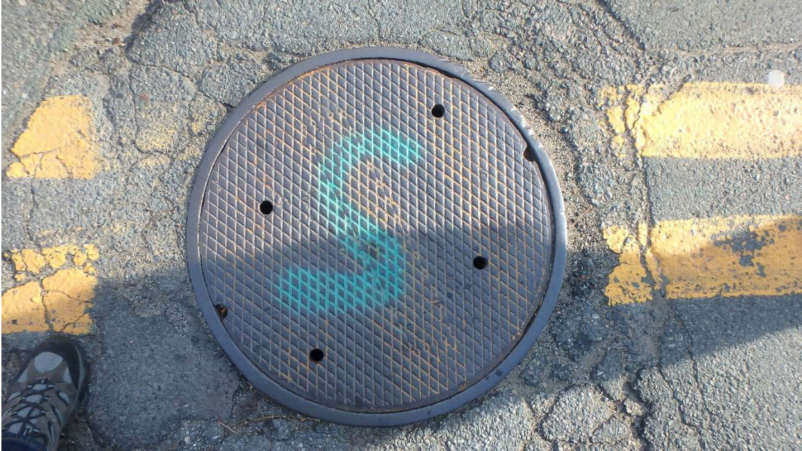
EXISTING MANHOLE MA-121 SHEET C-1 STATION 2+86 FRAME AND COVER PHOTO
