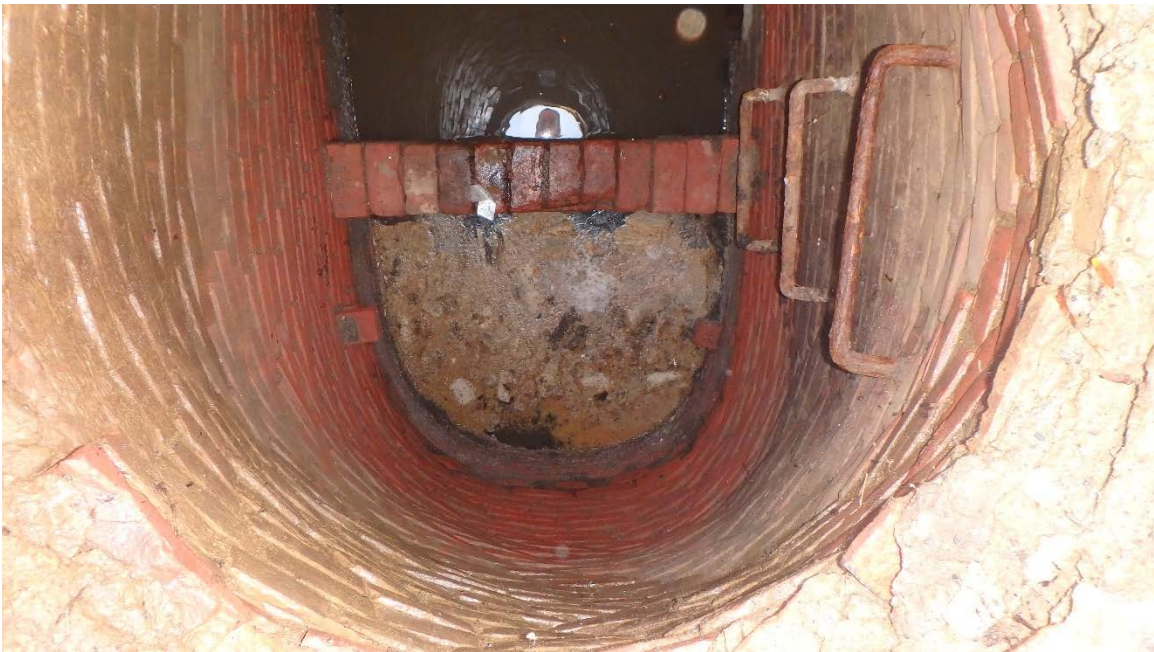
EXISTING MANHOLE MA-121 SHEET C-1 STATION 2+86 INTERNAL PHOTO #3
