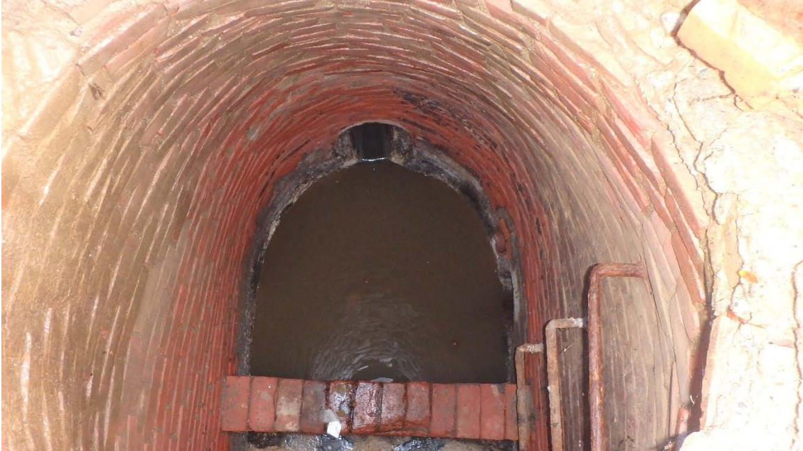
EXISTING MANHOLE MA-121 SHEET C-1 STATION 2+86 INTERNAL PHOTO #2
