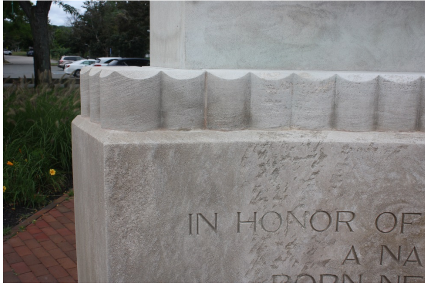
Picture 11 – Completed erosion restoration
