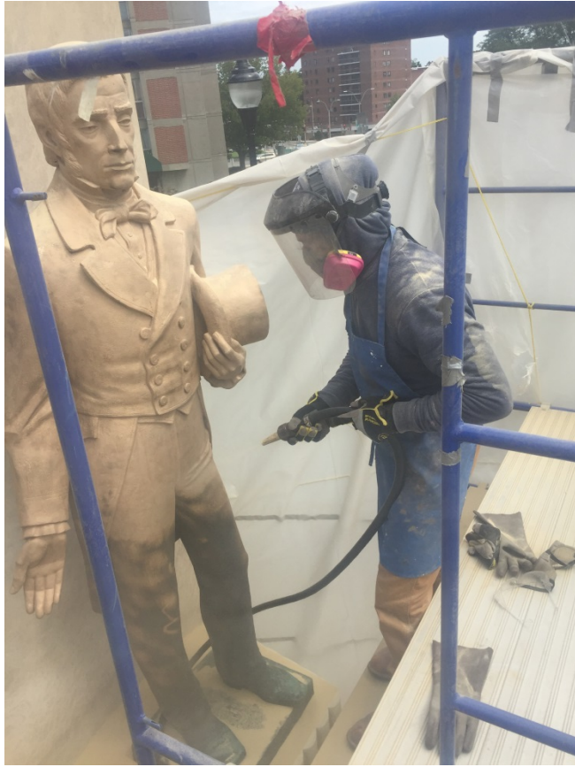
Picture 6 – Air blasting
