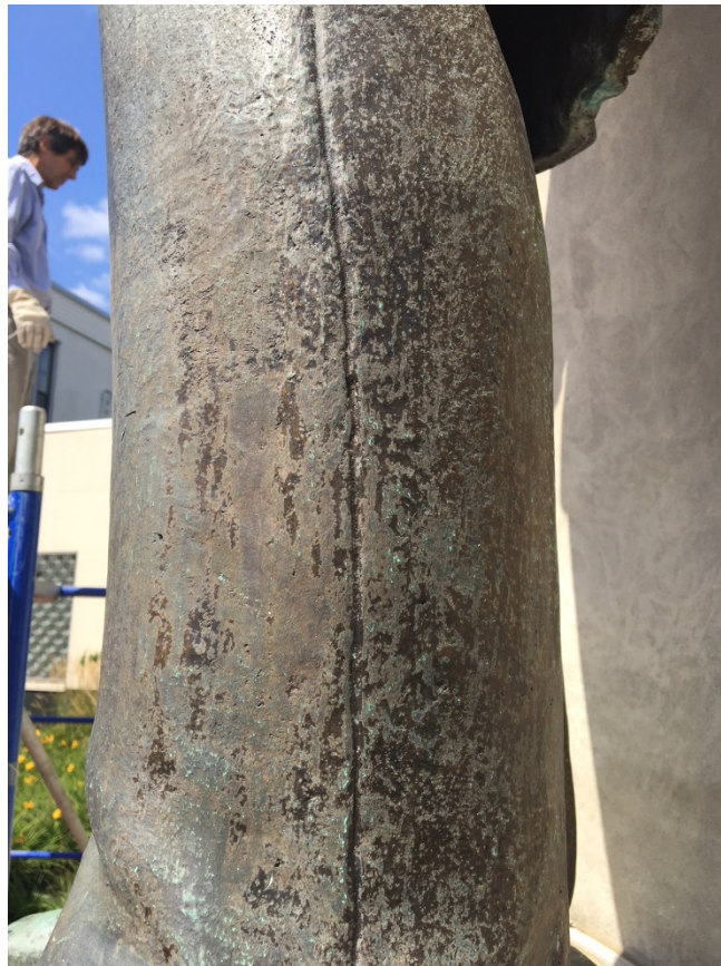
Picture 2 – Bronze corrosion
