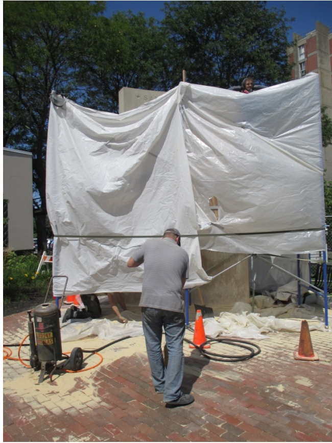
Picture 4 – Pipe staging
