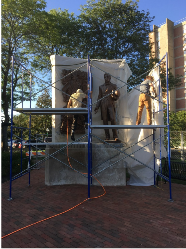
Picture 5 – Masking stone surfaces
