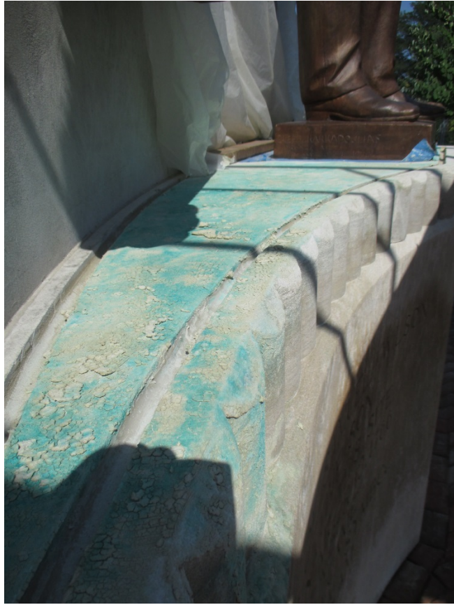
Picture 9 – Cleaning with poultice
