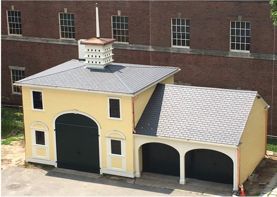
Photo of the Whittemore Robbins Carriage House immediately after CPA project completion in 2017. This image depicts the first town owned properties to go through rehabilitation utilization CPA funding.
