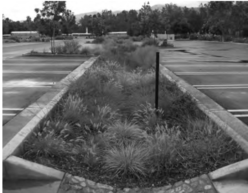
Bioswales reduce the heat island effect
