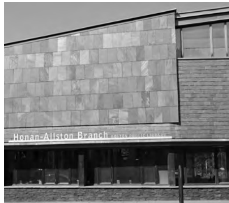
A variety of cladding materials
