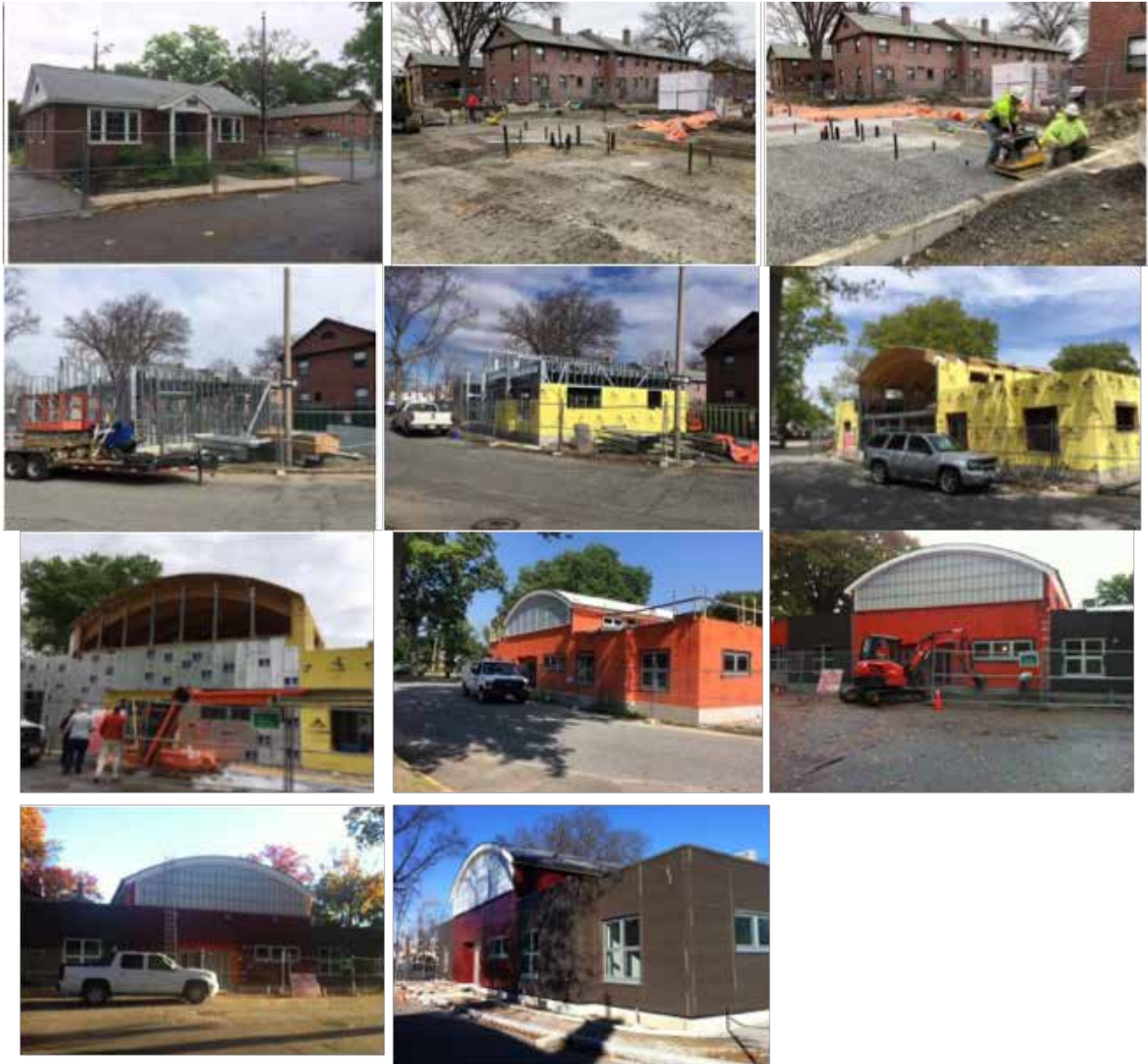
Progression photos of the construction of the Life and Skills Building.
