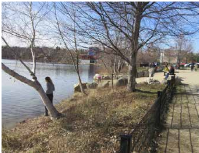
The Spy Pond Project includes pathway resurfacing and erosion control.
