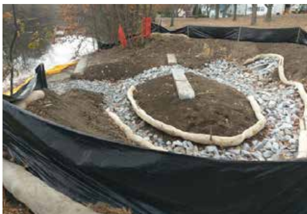
New stormwater infrastructure along the Mystic River.
