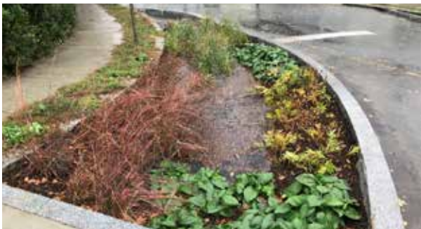
Completed bioretention basin (rain garden) filtering water during a rain storm at the intersection of Egerton and Herbert.
