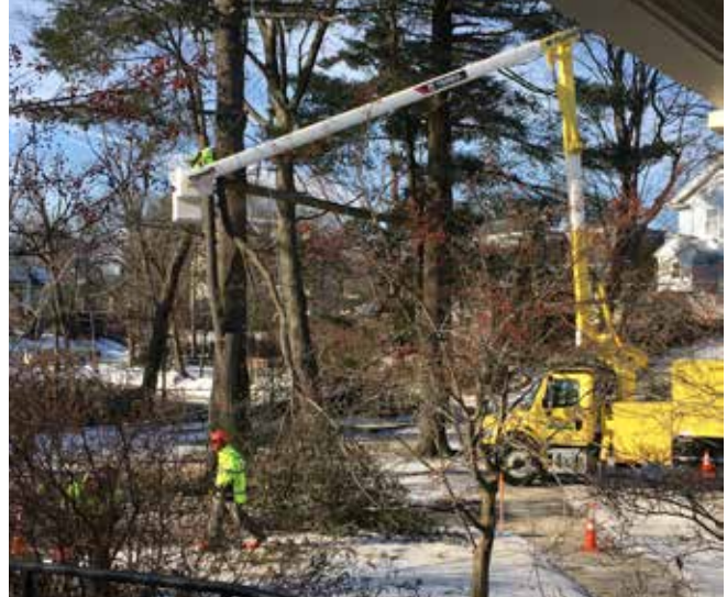
New bucket truck used by Forestry Division.
