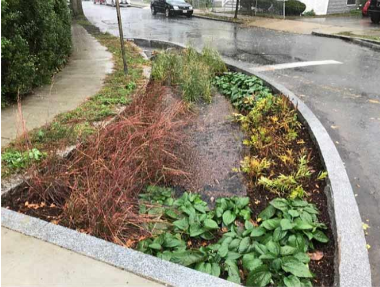
Green Infrastructure: Bioretention Basin construction at Egerton Rd/Herbert Rd, Arlington – September 2018
