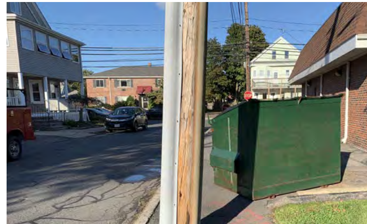
Figure 57. Residents need a more accommodating streetscape for pedestrian and bicycle safety.
