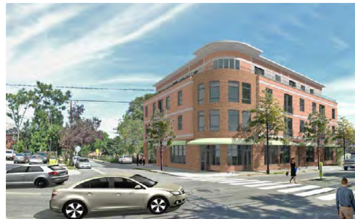
Figure 33. Recent redevelopment efforts on Broadway include the 117 Broadway project, which will add 14 affordable housing units with ground-level commercial space for the Arlington Food Pantry and an additional tenant.
