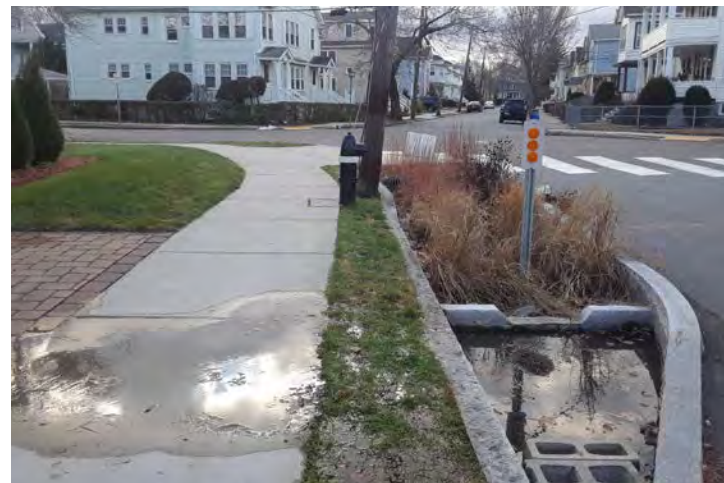
Figure 21. Green infrastructure, like this rain garden in East Arlington, could improve the street aesthetically and provide environmental services.
