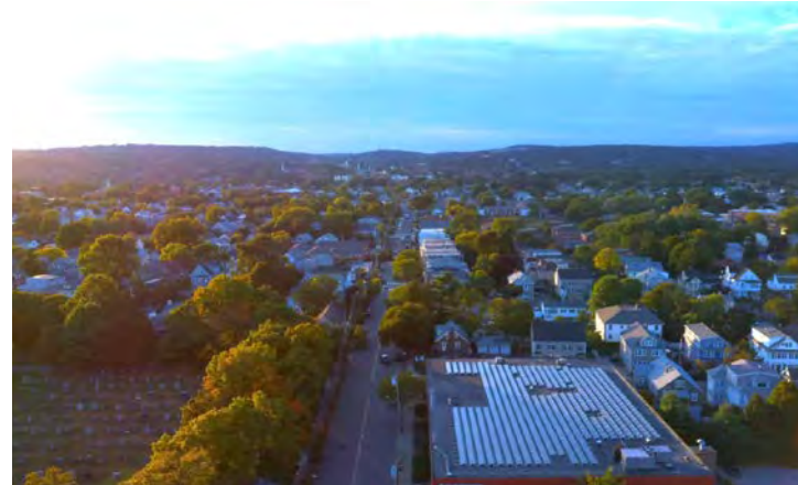
Figure 52. This planning study has highlighted the Lahey site, situated on the eastern extreme of the corridor, as a site with high potential for redevelopment.
