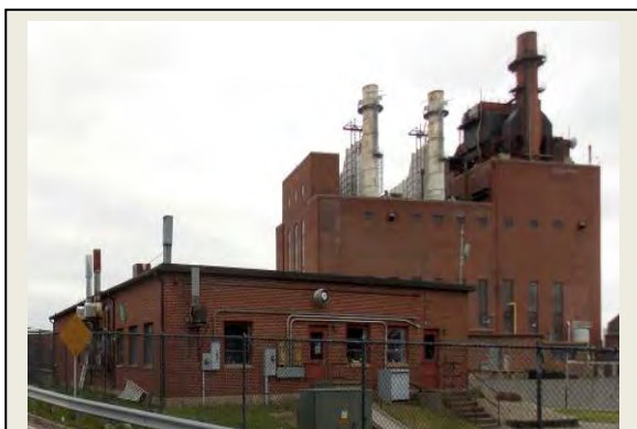
The West Springfield Generating Station (1947-49) was included in the historic resource survey update for West Springfield.
