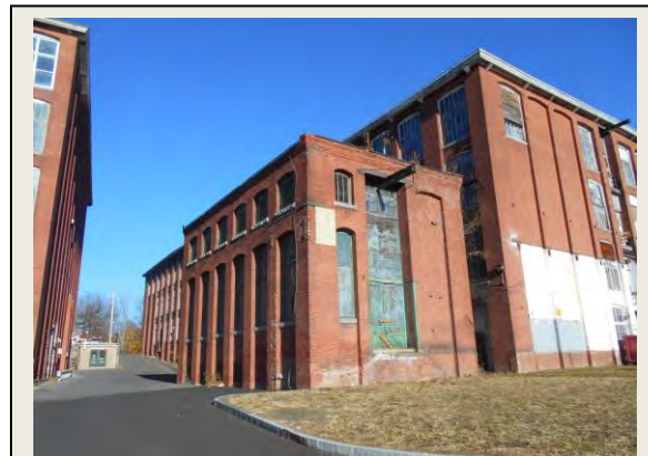
Former industrial buildings in Easthampton now include housing, offices, artist studios, restaurants, and an indoor playground.
