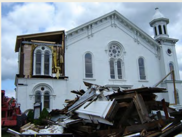
The tornado of 2011 damaged and destroyed many properties such as this one in the town of Monson.
