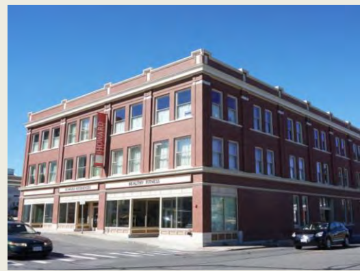
The rehabilitation of the Howard Building, Pittsfield.
