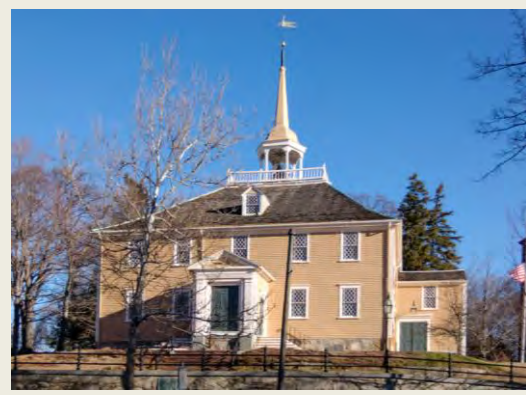
The Old Ship Meetinghouse, Hingham, following its restoration.
