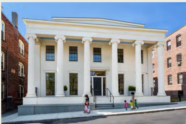
The rehabilitation of the Alvah Kittredge House by Historic Boston, Inc.
