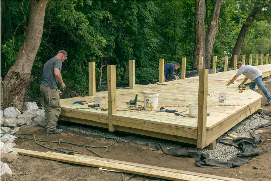
Installation and completion of the boardwalk, May-July 2019. Photo credit: David Mussina.
