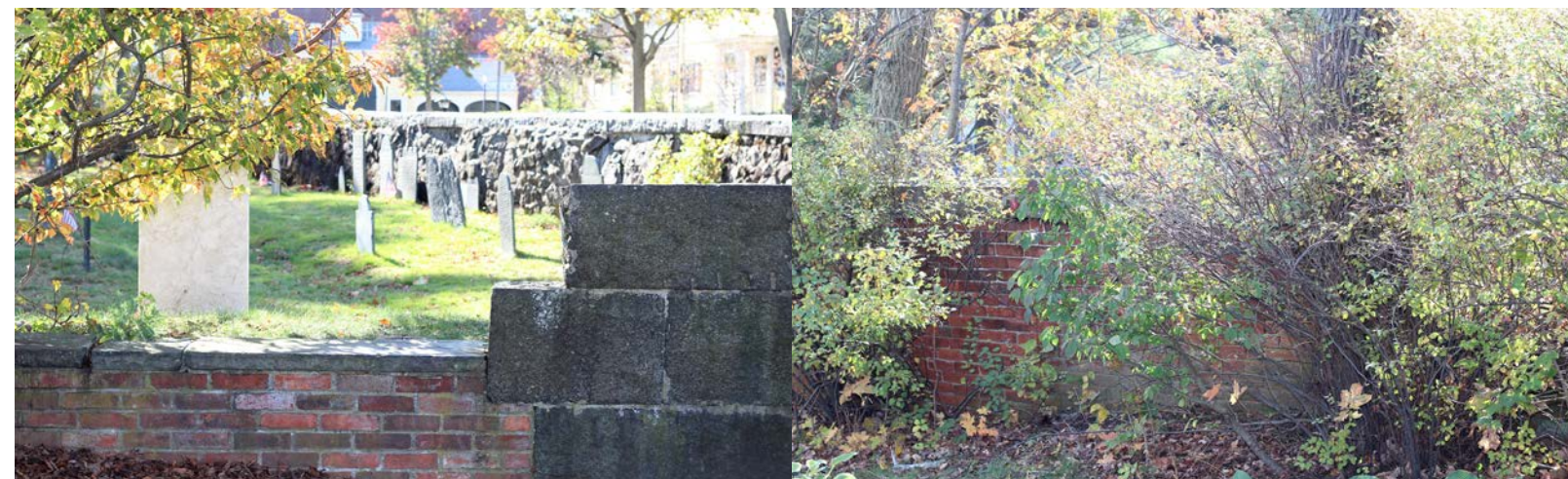
7. Northeast wall - brick
