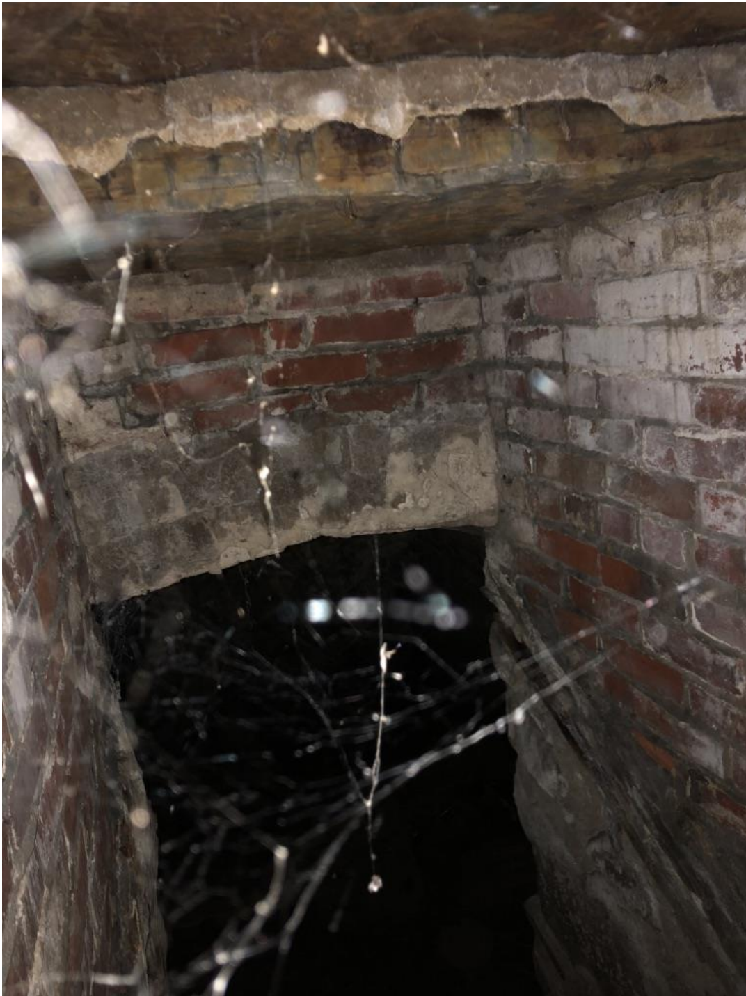
Photograph of interior of brick vaulted tomb on the norther edge of the burying ground. The photograph shows the small granite roofed entry chamber in the foreground and the brick vaulted burial chamber in the background. The burial chambers of the four tombs at the northern edge of the burying ground are deeper than the single chamber on the western edge.
