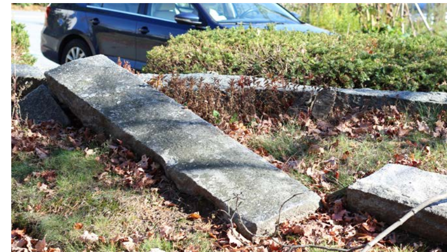
5. Coping stones lying next to wall
