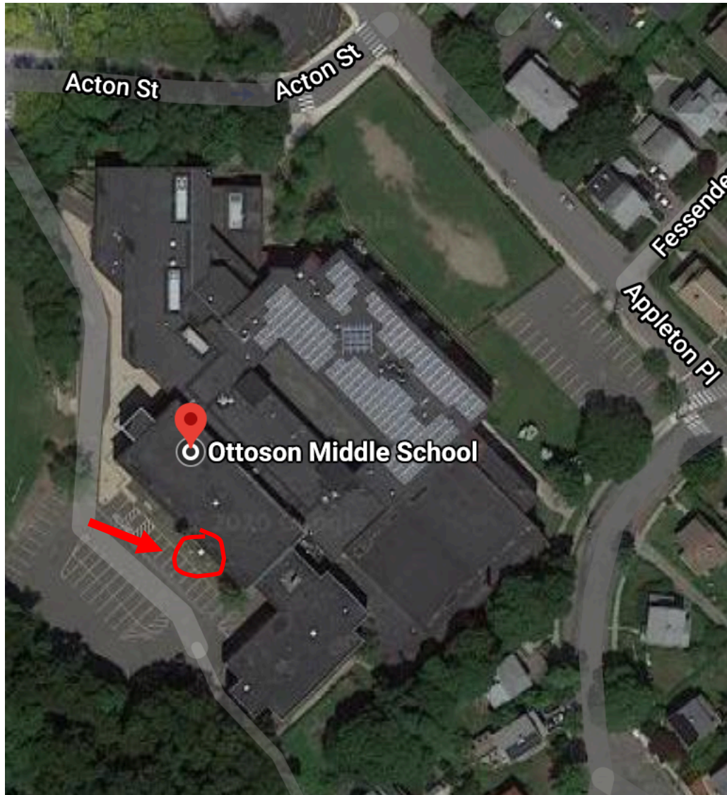
Ottoson Middle School: 63 Acton Street The textile bin is located off the upper staff parking lot off Acton Street
