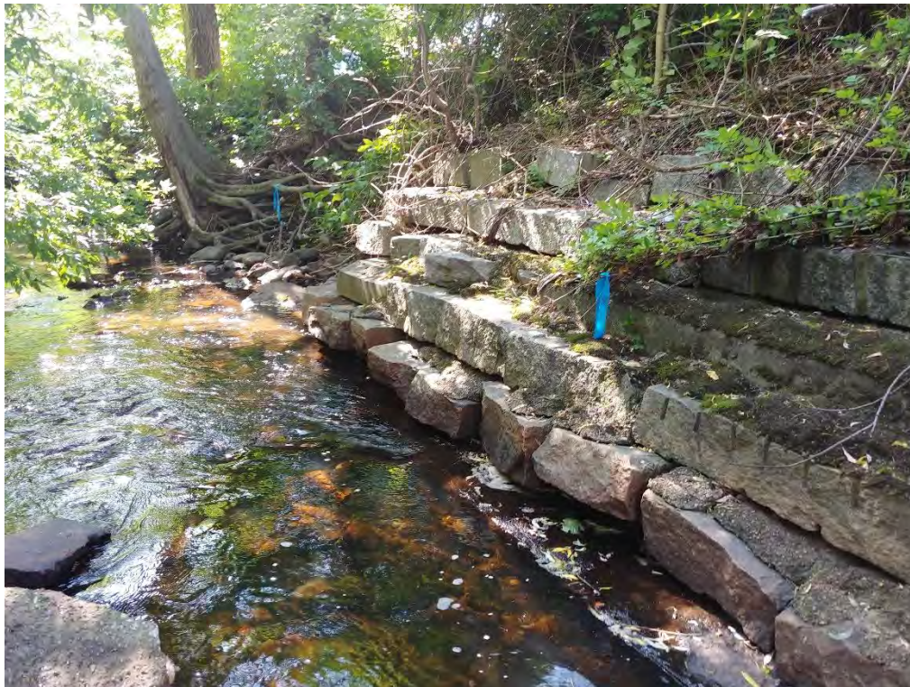
Photo 3. View of stone wall bank, looking southeast near flag A-11 .
