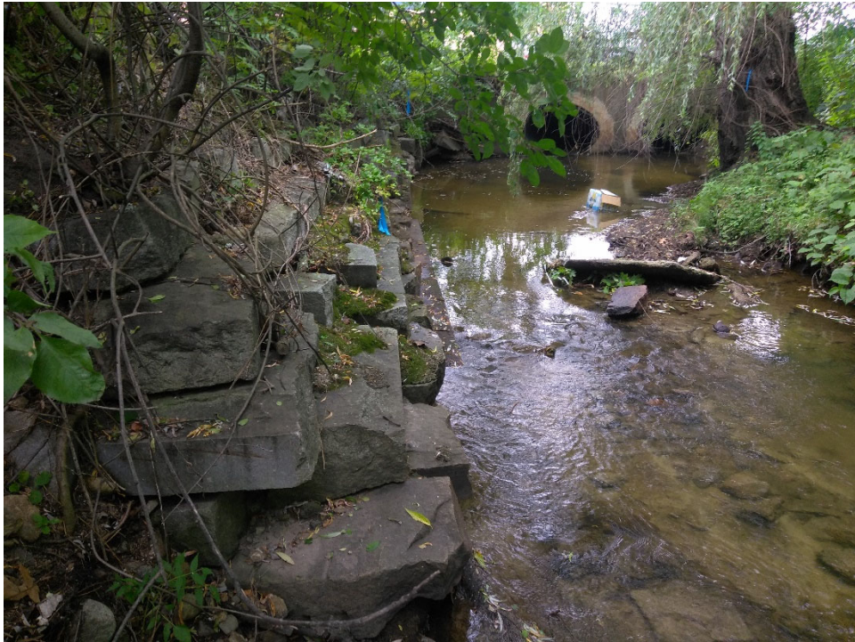
PICTURE 9: MILL BROOK AT EAST HEADWALL
