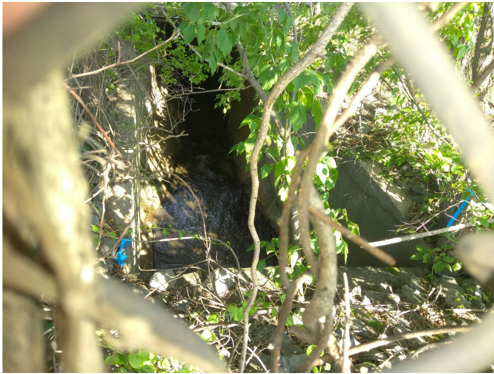
PICTURE 3: CULVERT HEADWALL WEST SIDE OF SITE
