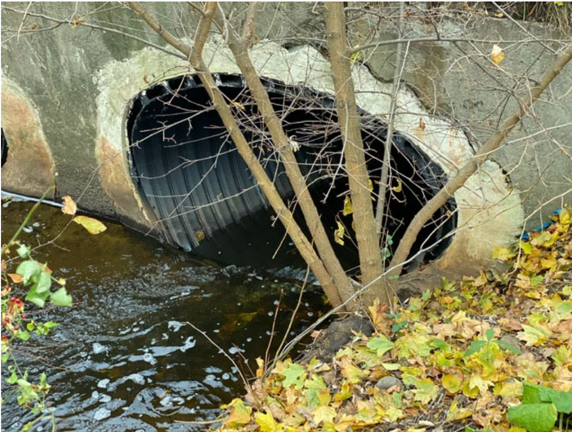
PICTURE 2: CULVERT HEADWALL EAST SIDE OF SITE
