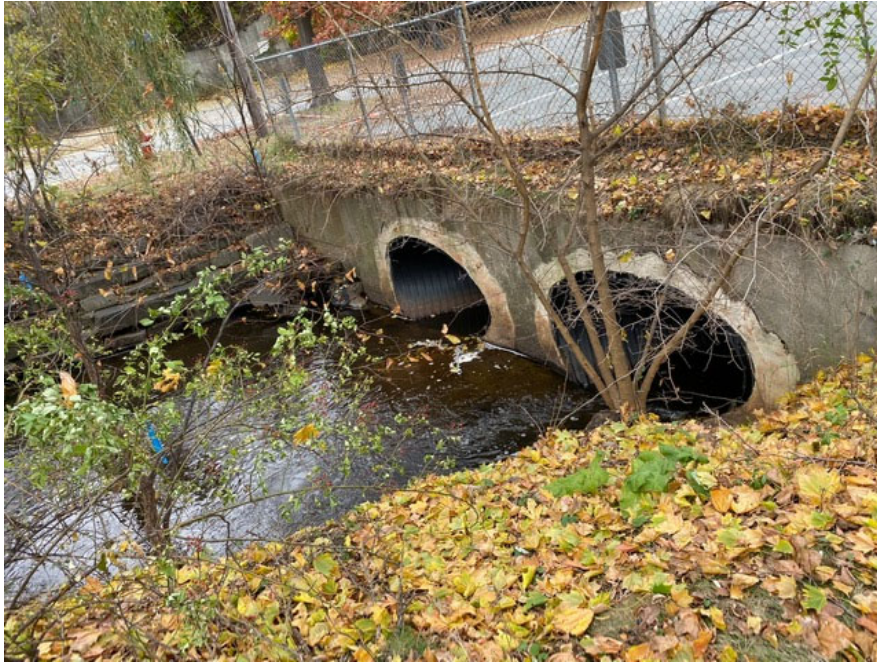
PICTURE 1: CULVERT HEADWALL EAST SIDE OF SITE
