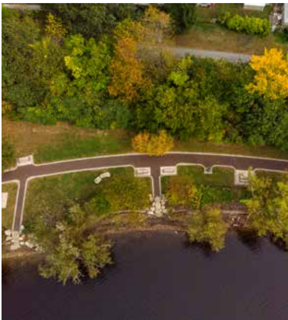
Pathway at Spy Pond Park, part of the Spy Pond Park Stabilization Project.
