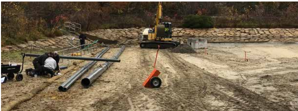
Phase 1 work at Arlington Reservoir
