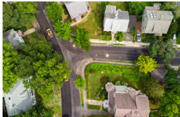
Pavement preservation operation in Arlington Heights
