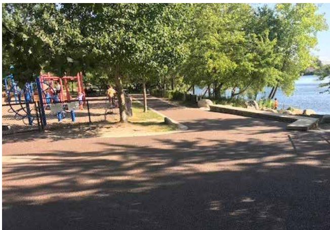
The Spy Pond Project included resurfacing the pathway with an ADA accessible porous pavement.
