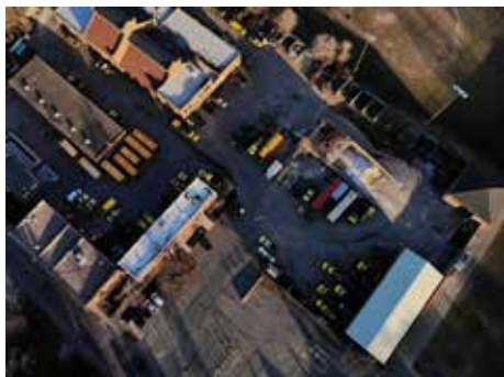
From above, DPW Yard at 51 Grove Street
