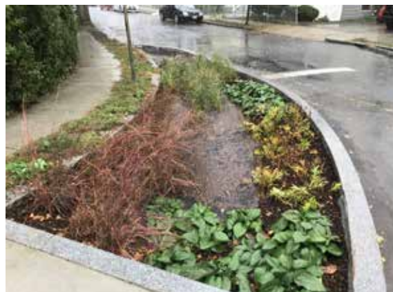
A rain garden in East Arlington is vegetated with native plants. Rain gardens slow down stormwater runoff and remove pollutants before the stormwater enters the municipal stormwater system and travels to a water body, like Alewife Brook. Photo Patrick Herron, MyRWA.
