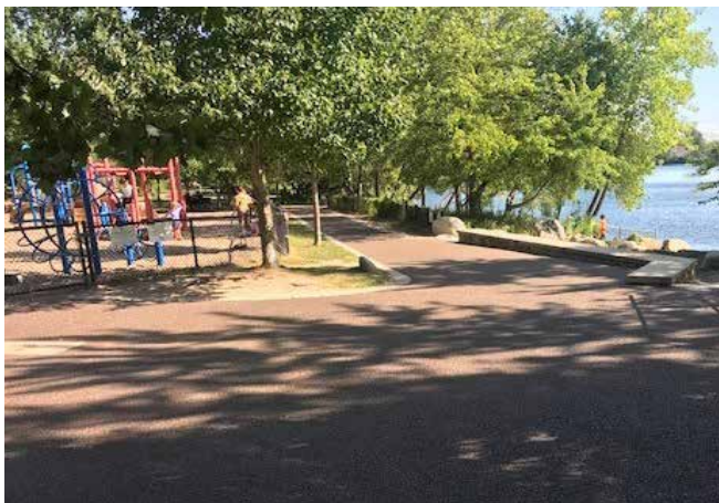
The Spy Pond Project included resurfacing the pathway with an ADA accessible porous pavement.
