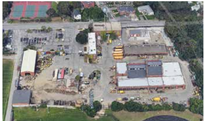
Overview of DPW Town Yard
