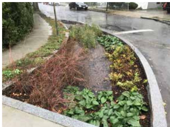
A rain garden in East Arlington is vegetated with native plants. Rain gardens slow down stormwater runoff and remove pollutants before the stormwater enters the municipal stormwater system and travels to a water body, like Alewife Brook. Photo Patrick Herron, MyRWA.
