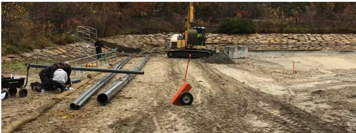
Phase 1 work at Arlington Reservoir
