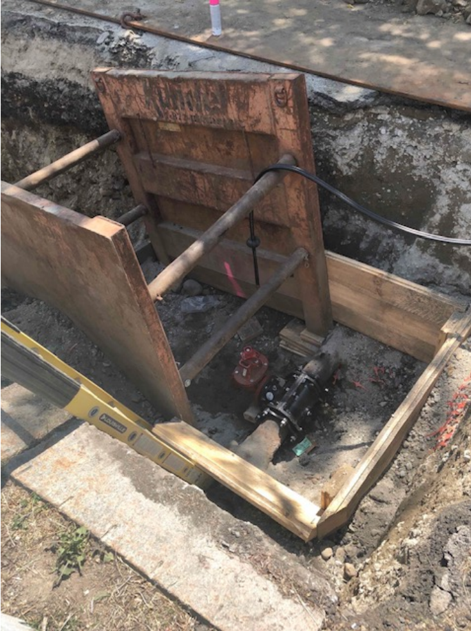
Photograph 1: Installation of a new temporary water line to the high school (6/4/20)
