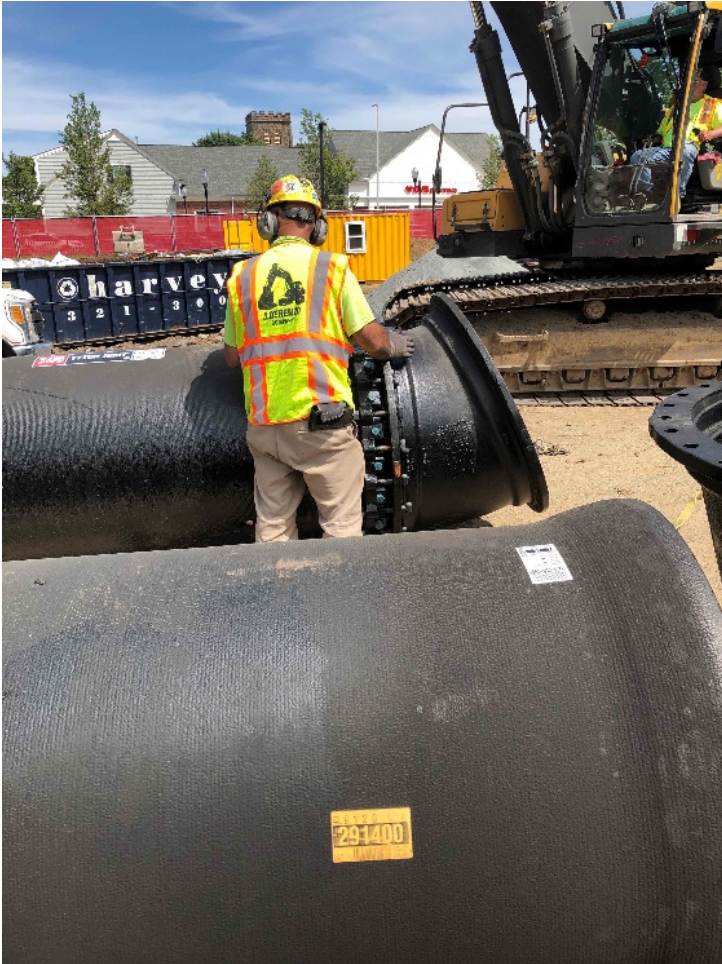
Photograph 1: Derenzo assembling 36in drain-pipe for installation in the front lawn area (6/15/20)
