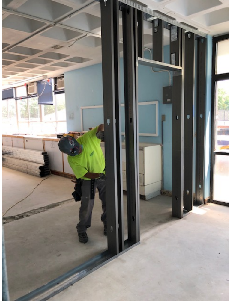
Photograph 4: TJ McCartney framing in the transaction window in Downs building (6/26/20)
