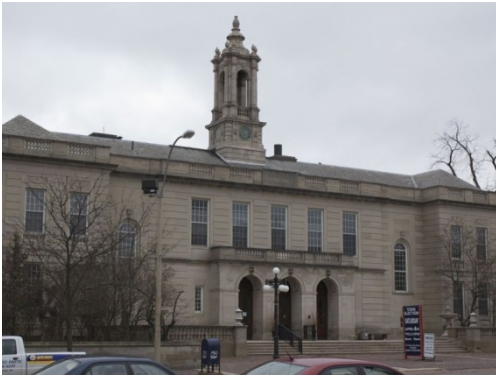
Town Hall + Annex
