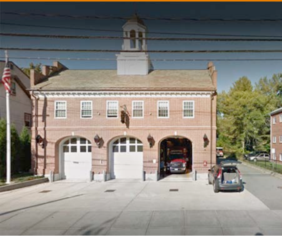
Highland Fire Station
