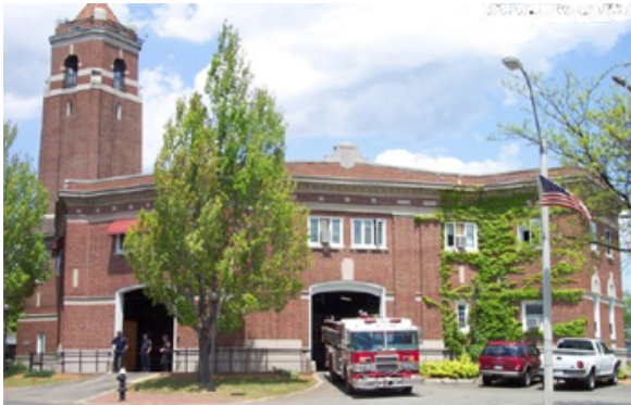
Fire Department Facilities
