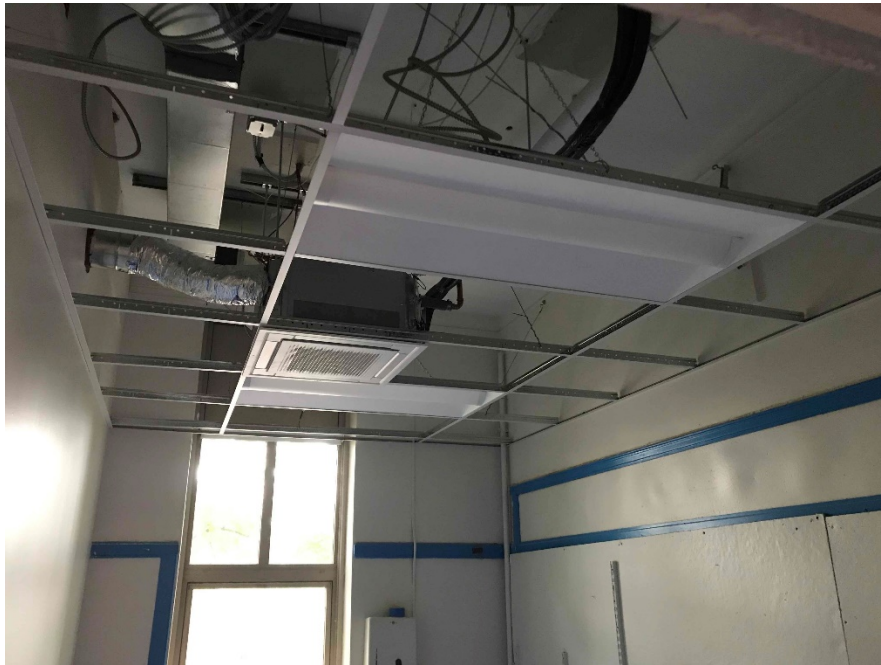
Photograph 3: Ceilings framed and installation of finishes underway
