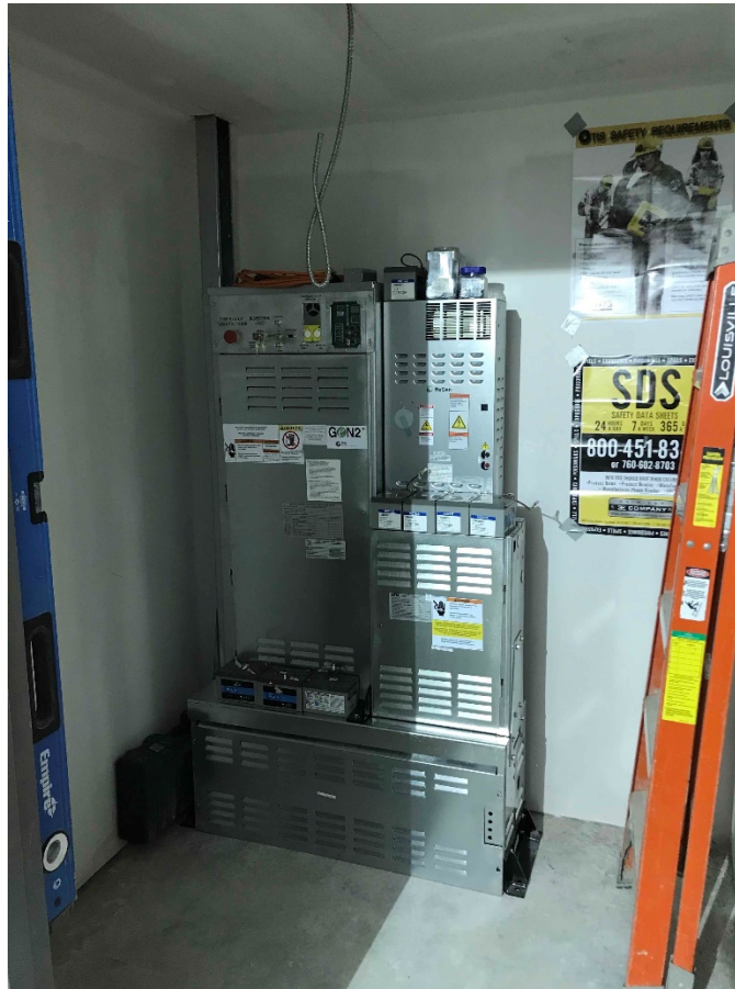
Photograph 7: Elevator controller installed
