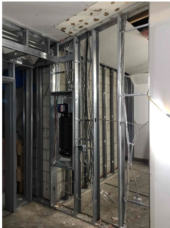
Photograph 2: Framing and electrical tie-in on 4 th Floor
