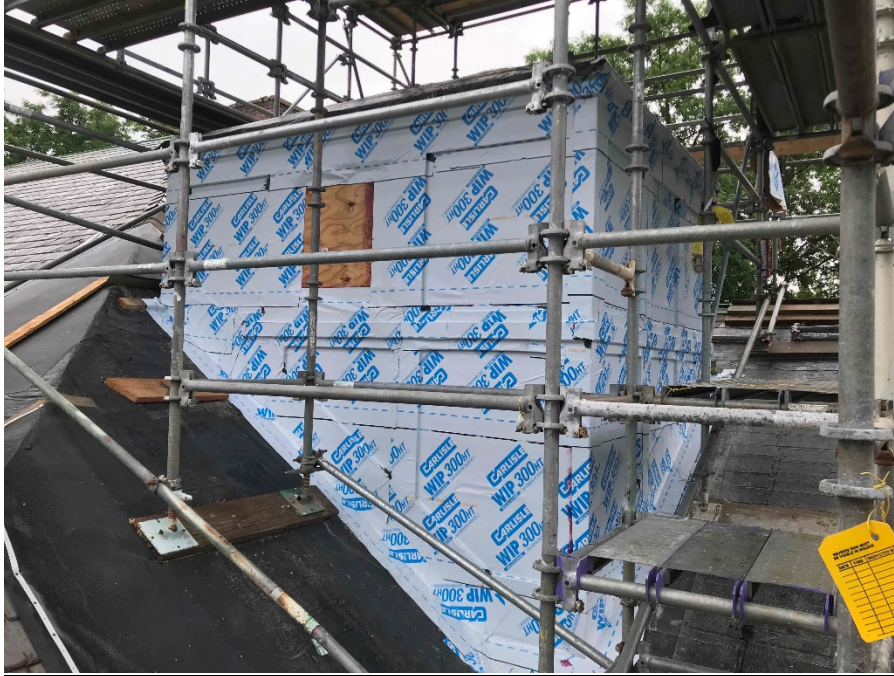
Photograph 1: Roofing underlay complete on top floor
