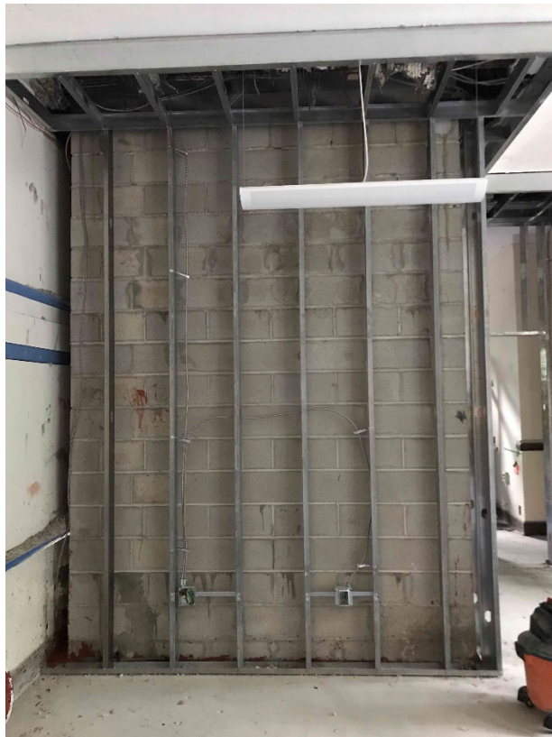
Photograph 4: Framing and mechanical, electrical, and plumbing (MEP) completed around CMU
