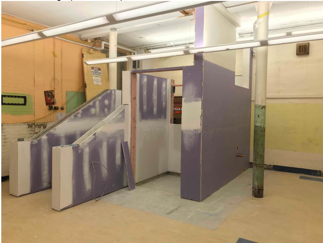
Photograph 6: Handicap lift drywall completed
