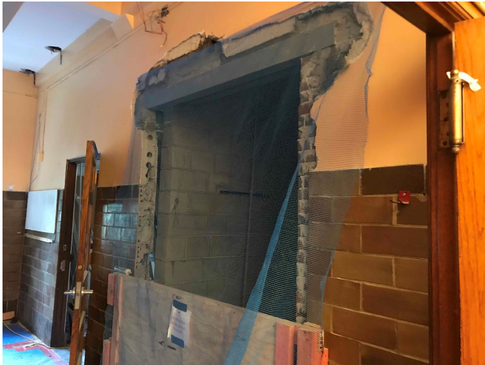
Photograph 5: Mesh protection at shaft for elevator installation
