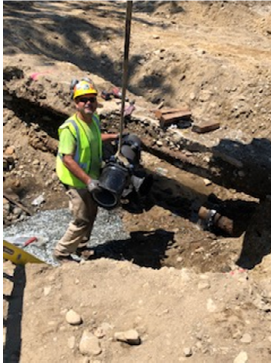
Photograph 1: Derenzo Installing 8in Water Line in Front Lawn
