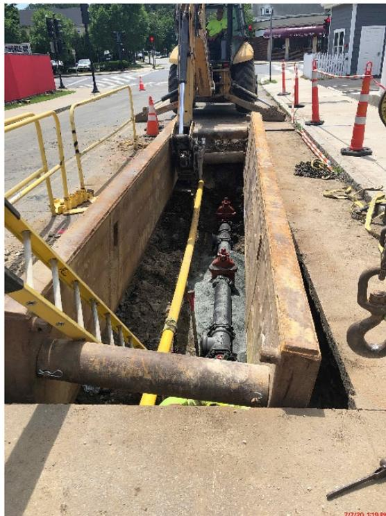
*Photograph 2: Derenzo working on water tie from schooler court to water line running along Mass Ave in front lawn*
