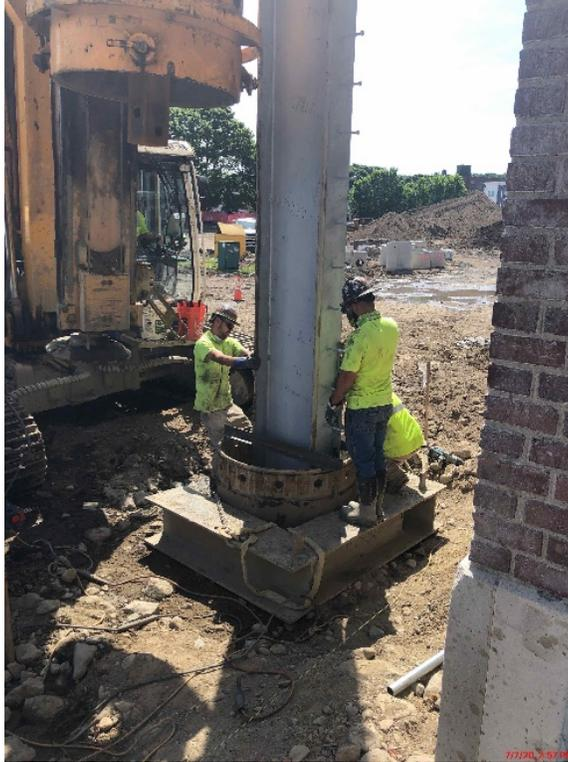
*Photograph 1: Keller North America setting beams for SOE along the front of the Auditorium building*
