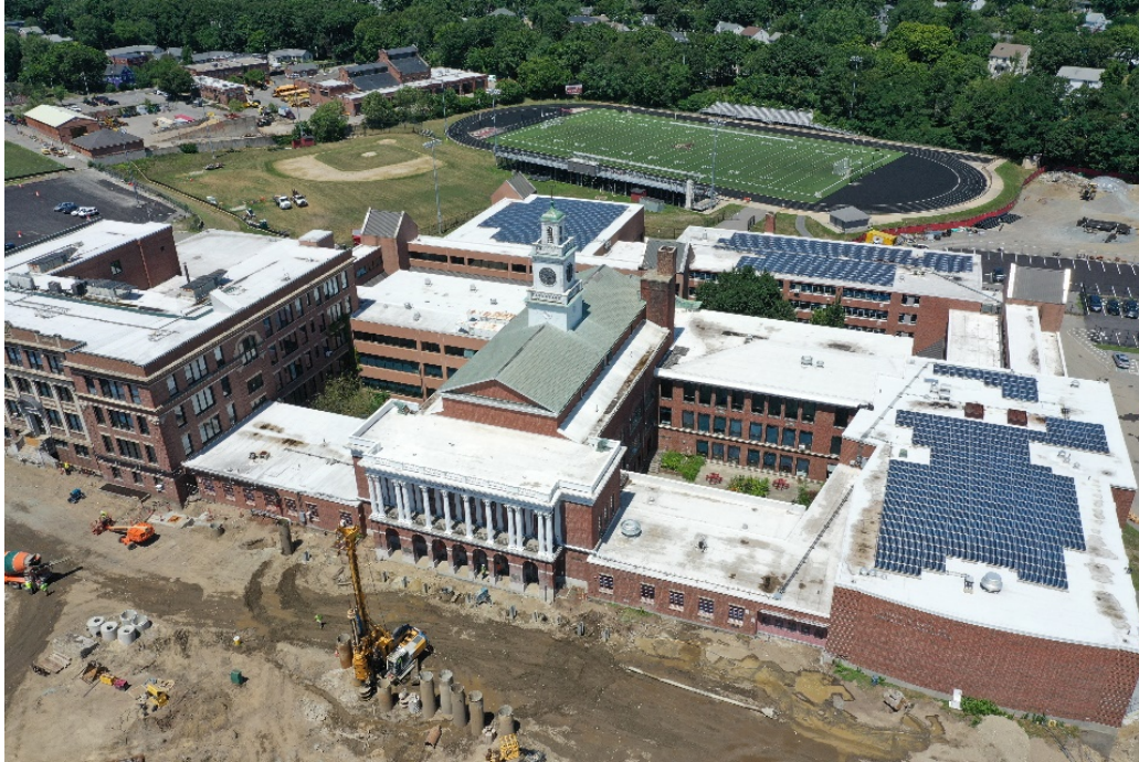
Photograph 1: Overview of Mass Ave Front Lawn Activities (From Drone)
