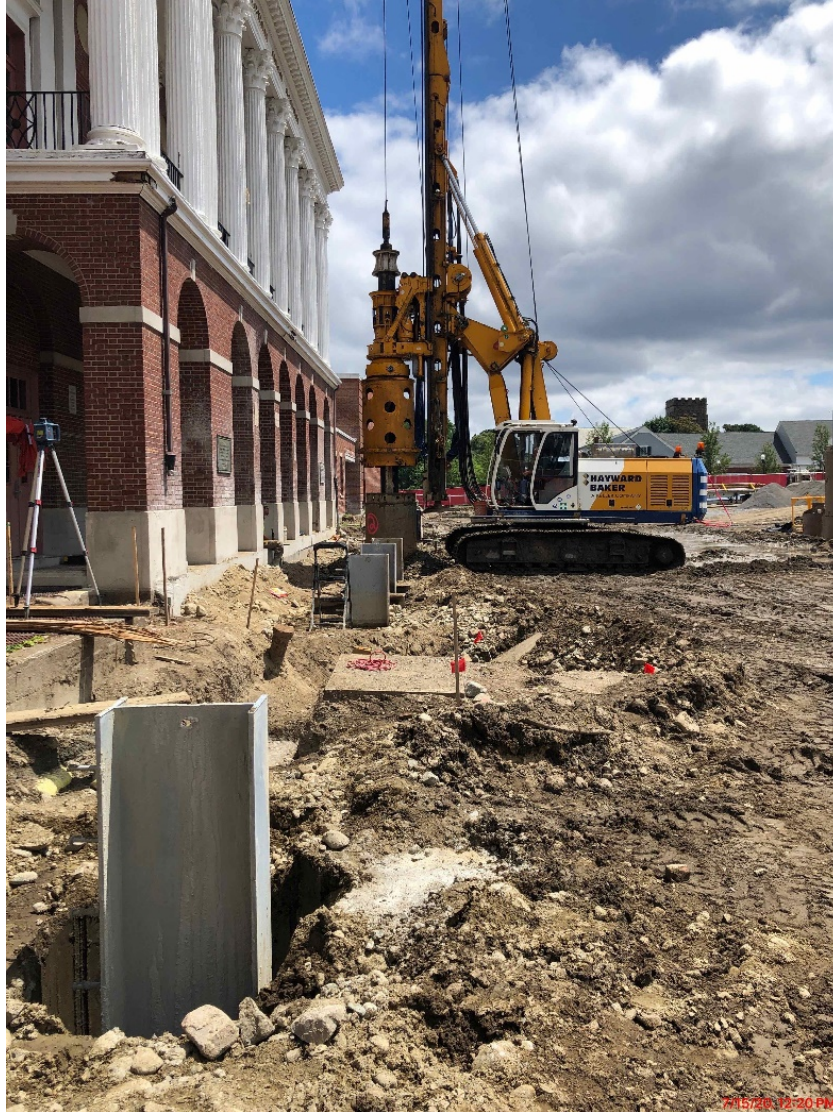
Photograph 5: Pile Installation at Mass Ave Front Lawn
