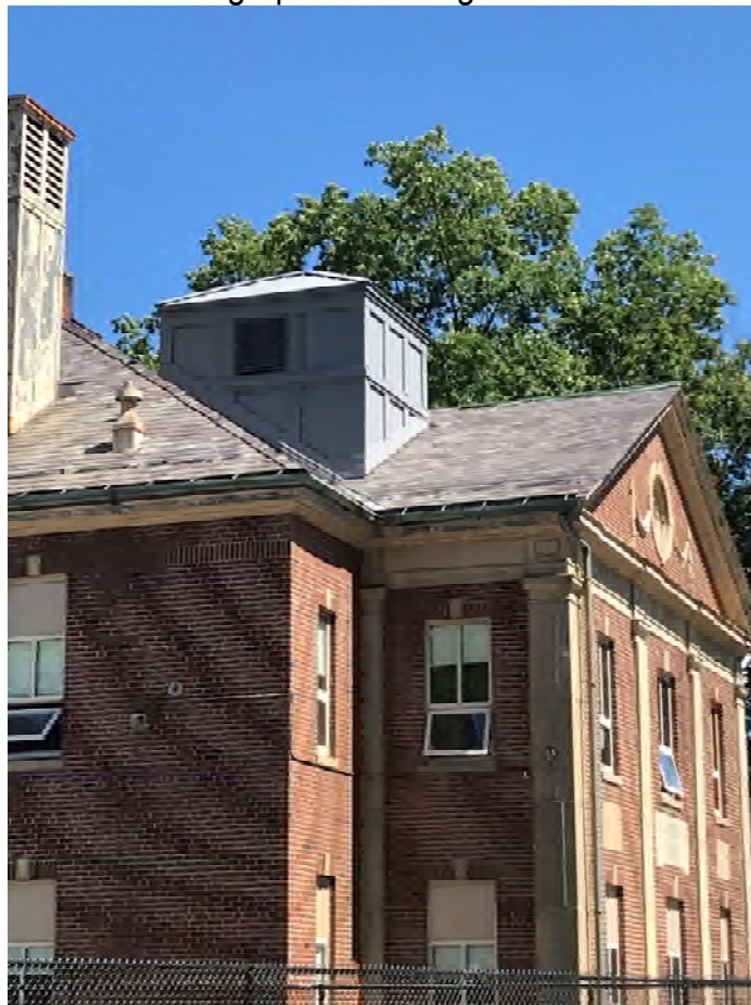
Photograph 10: New elevator shaft with temporary access stair tower removed
