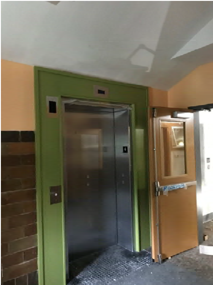
Photograph 5: New finished elevator on 4 th Floor
