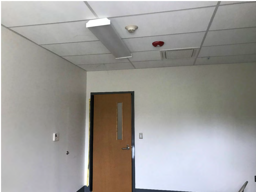
Photograph 2: Finished space on 4 th floor
