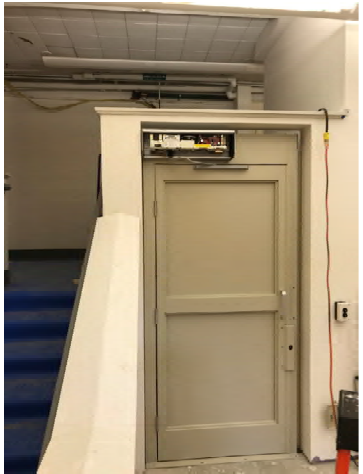
Photograph 6: ADA lift Installation
