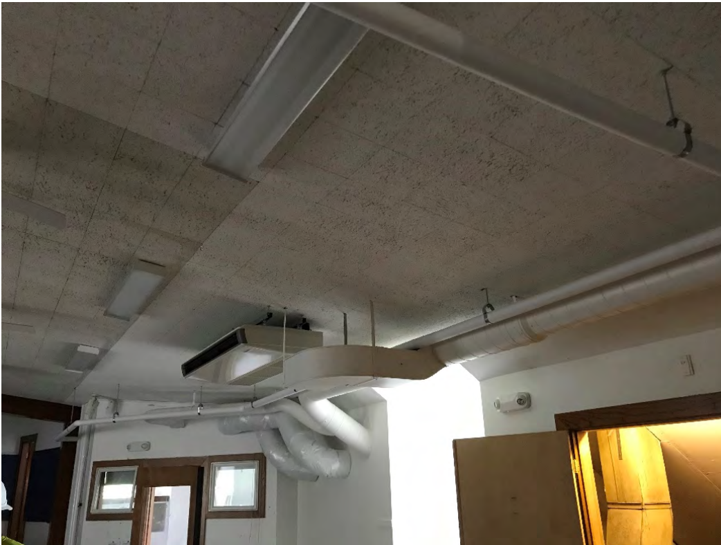
Photograph 3: New ductwork on 4 th floor
