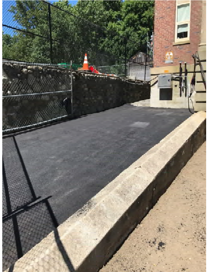
Photograph 8: New asphalt paving at front entry
