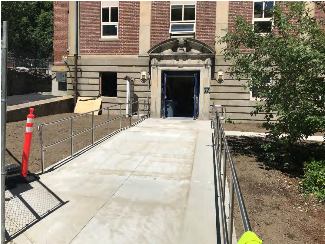
Photograph 4: New handrails and sidewalks at front entrance
