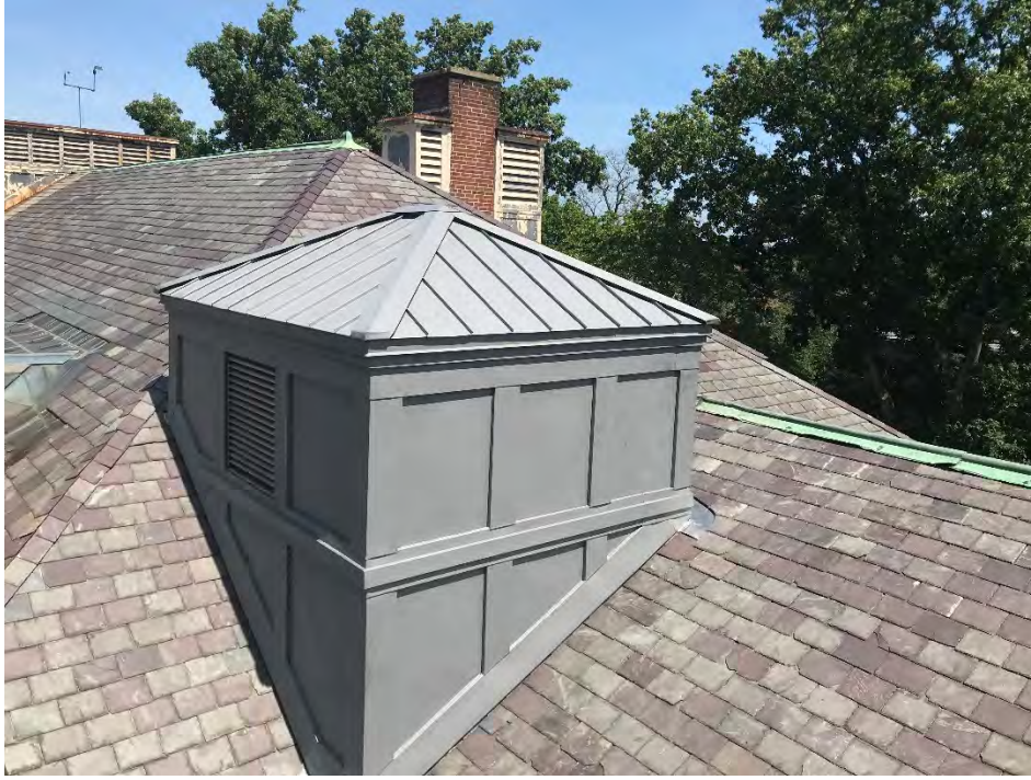
Photograph 1: Elevator shaft metal panels and roof slate installed
