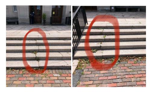
**Response:** The Contractor shall mark the four chipped stair treads and stockpile them for reinstallation. These treads shall be switched with treads located against either cheek wall such that the cracked corners are located
