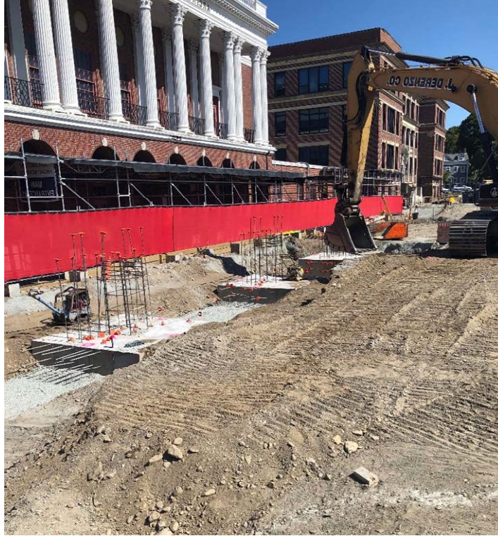
Photograph 1: Derenzo excavating continuous footings for the Phase 1 new building
