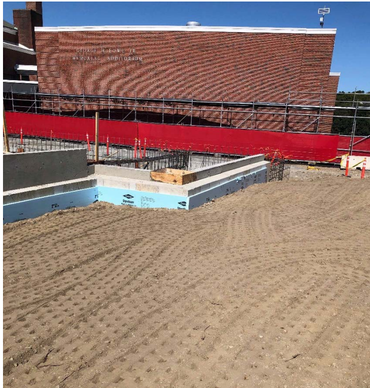
Photograph 2: Derenzo backfilling eastern foundation wall for Phase 1 new building
