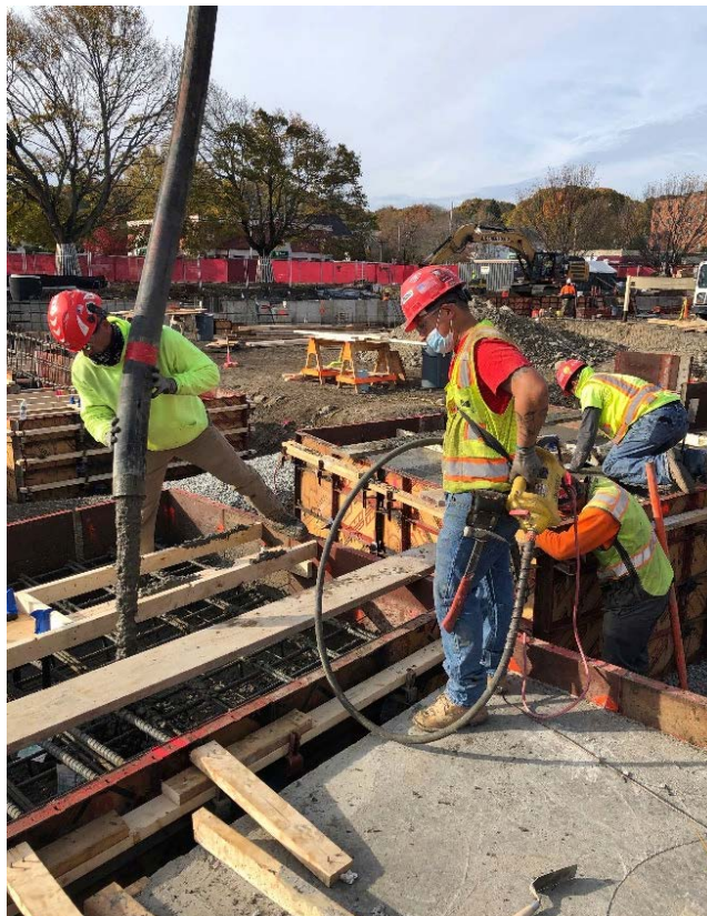
Photograph 2: Riggs Placing concrete for Phase 1 New Building footings
