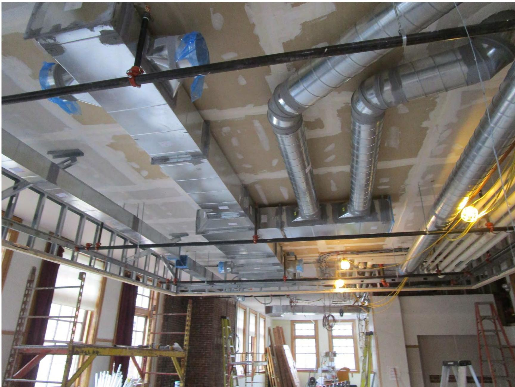
Ceiling patch, new ductwork, and soffit framing in Multi-Purpose Room
