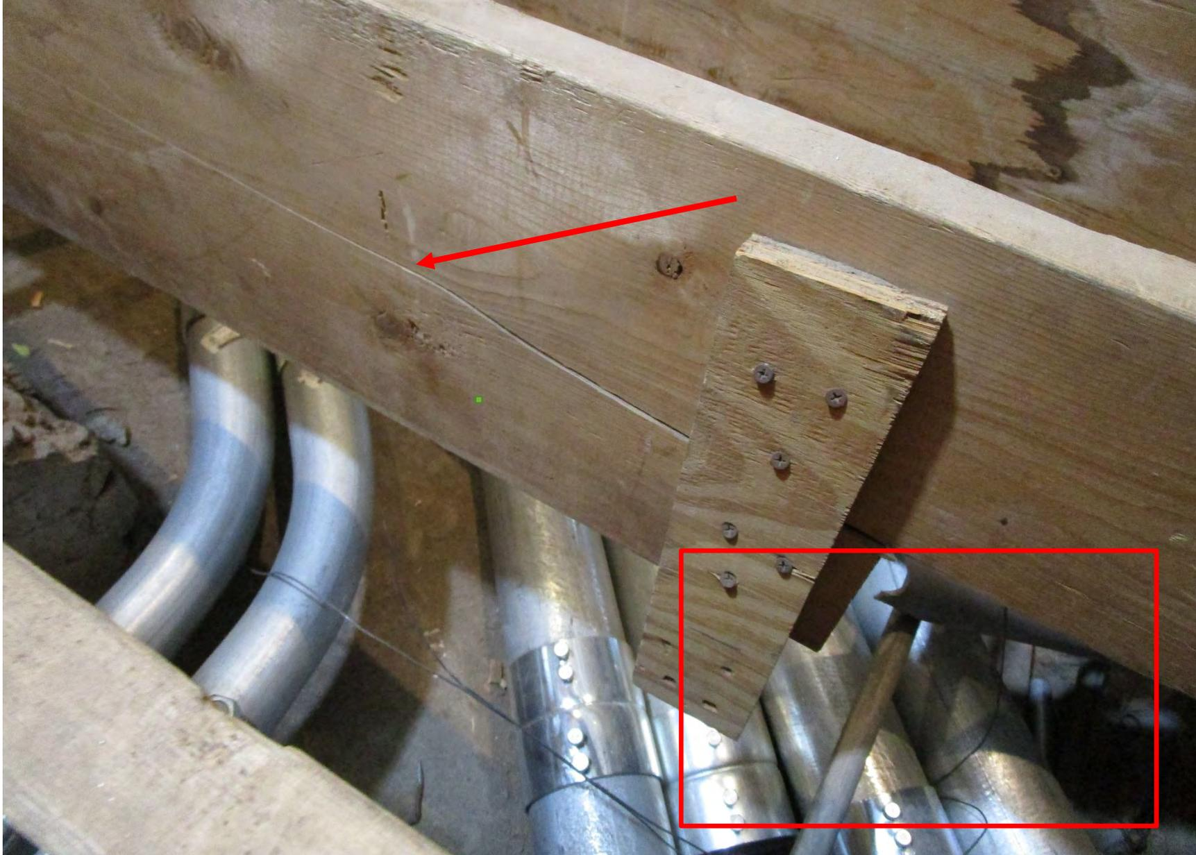
**Raised floor joist with existing check and cutout requiring repair.**
