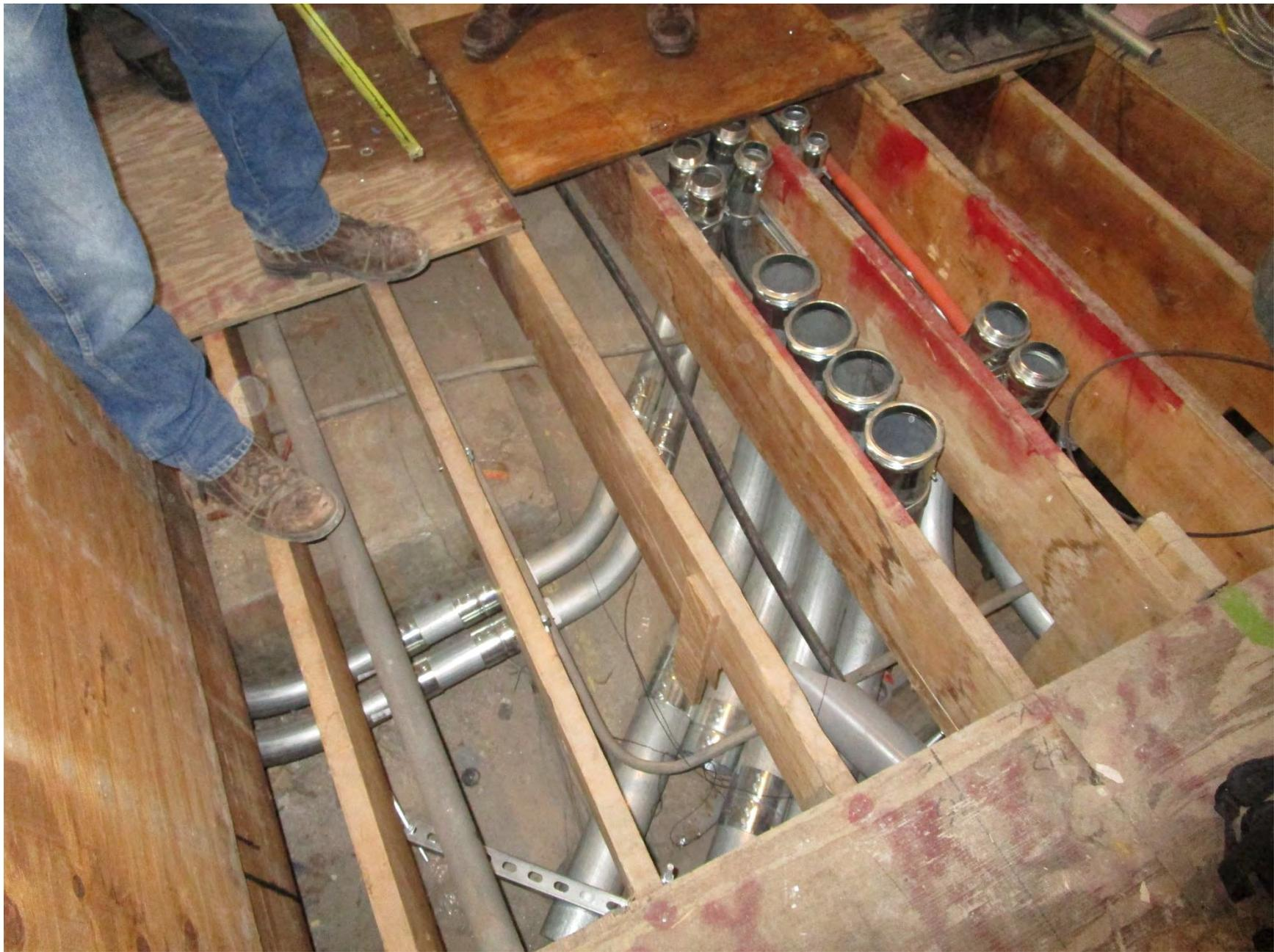
Boiler room raised floor with new switchgear conduit in revised location
