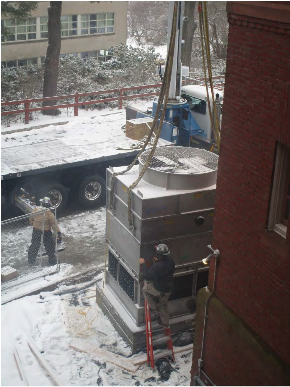
Rigging cooling tower on pad with truck crane
