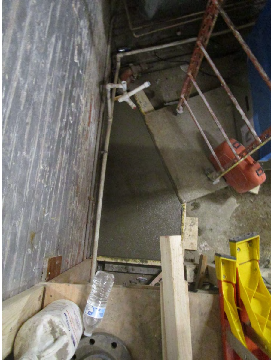
Mechanical room HV unit housekeeping pad extension
