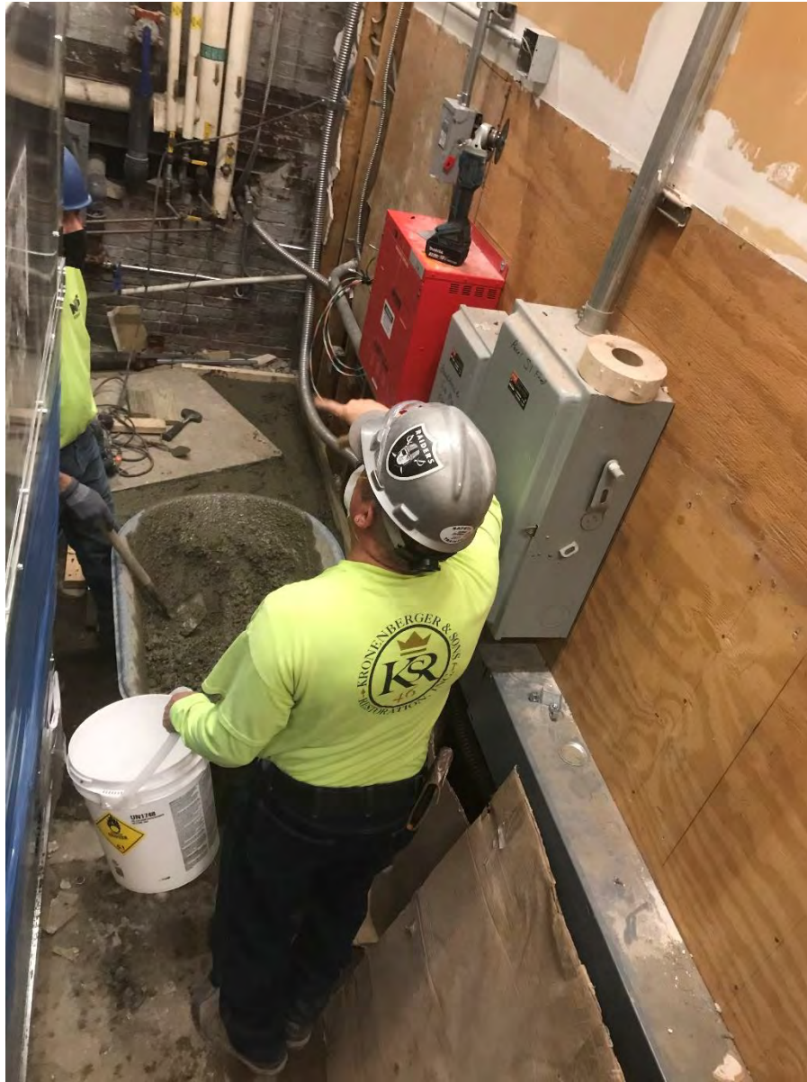
Mechanical room HV unit housekeeping pad extension
