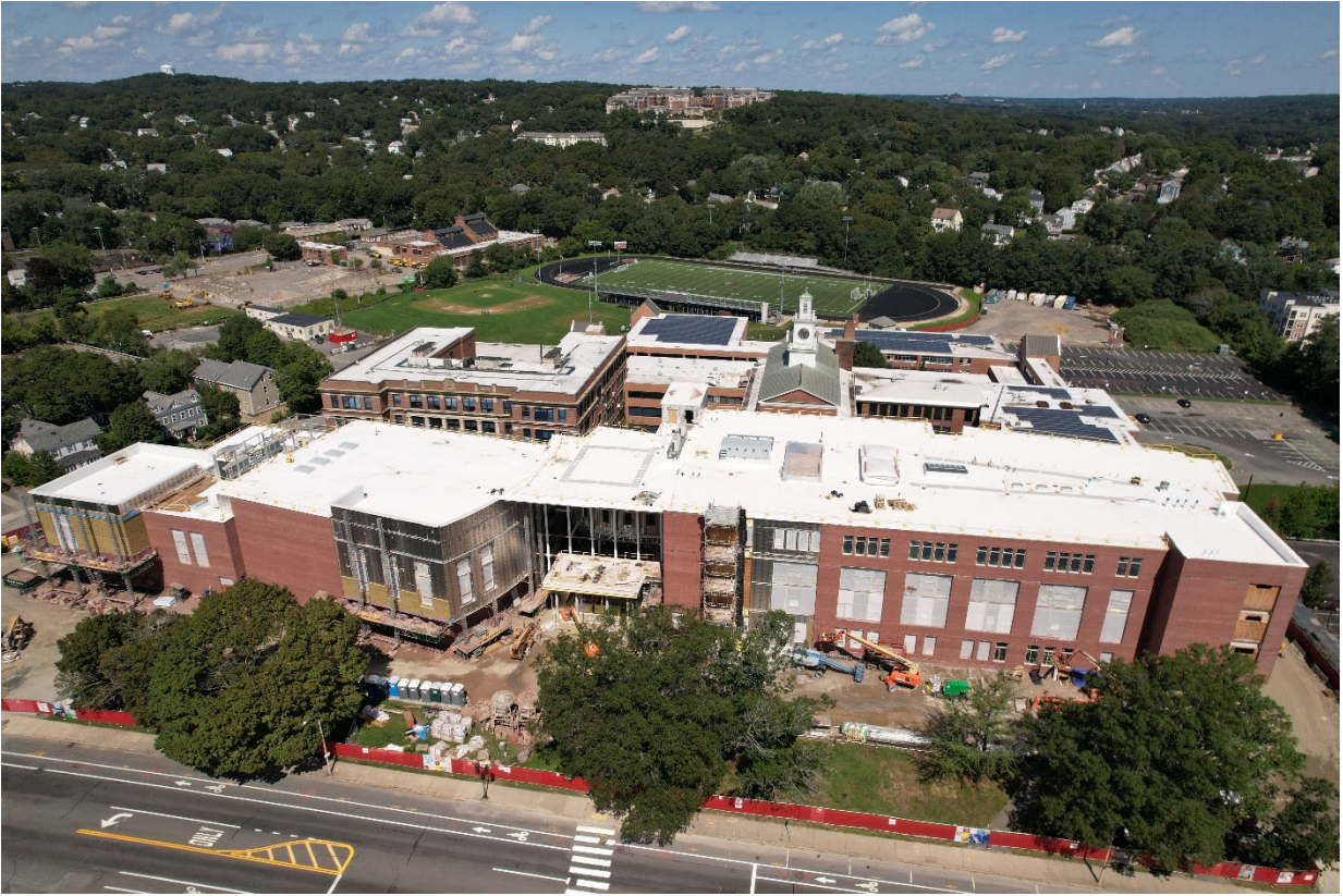
Arlington High School Building Project in progress
