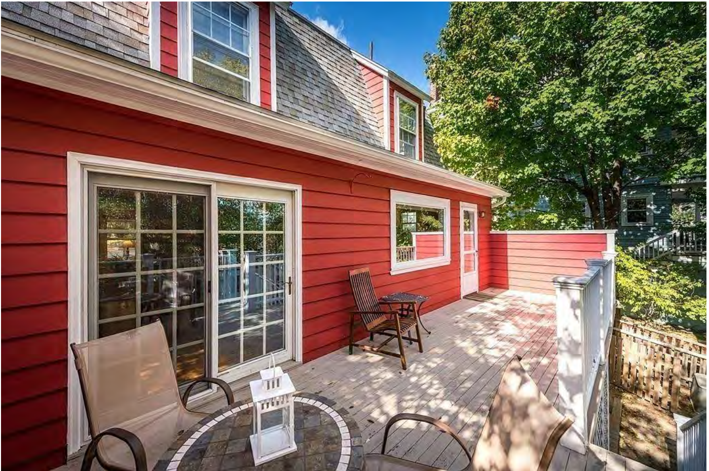
Rear deck – to be repaired and far section to be enclosed
