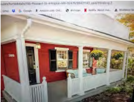
188P Front Porch w Railing photo2.jpg
