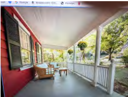
188P Front Porch w Railing photo1.jpg 4031K
