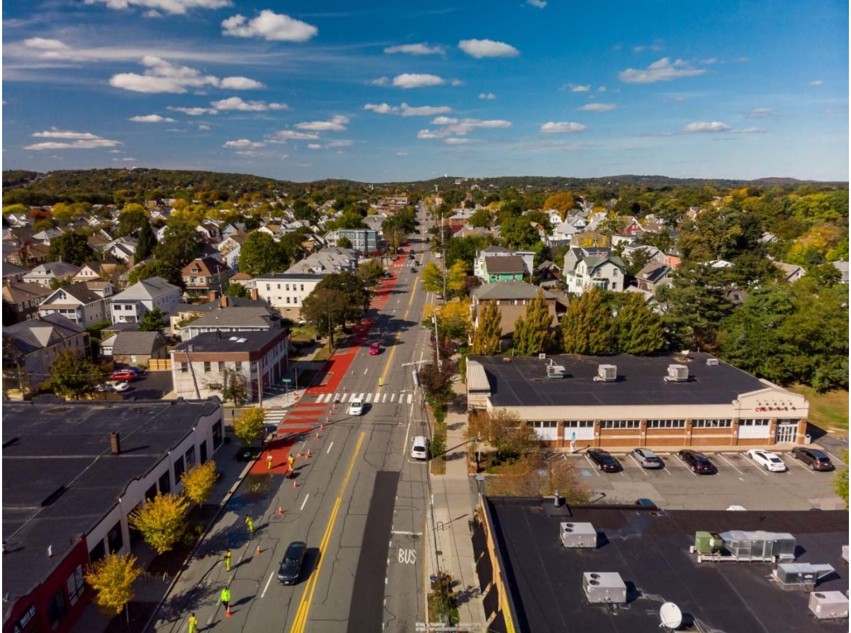
Priority Bus Lane Installation on Mass Avenue East
