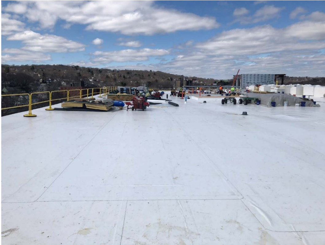
Photograph 3: Building D Roof
