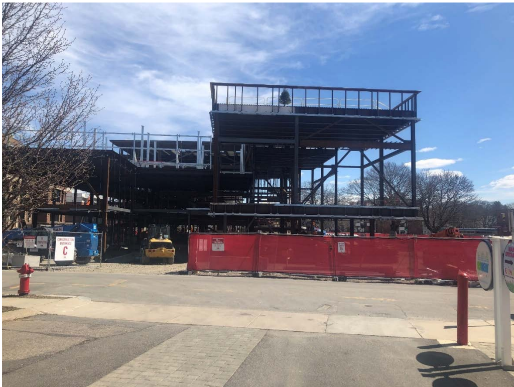
Photograph 2: Phase 1 Progress Photo from Schouler Ct.
