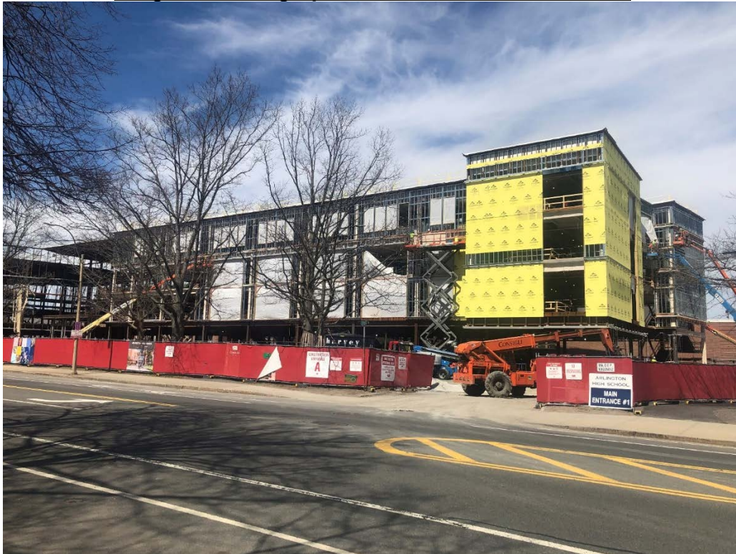
Photograph 1: Phase 1 Progress Photo from Mass Ave.
