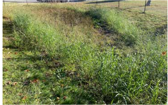
The Spy Pond Project included constructing a biobasin next to Scannell Field to improve stormwater quality before entering Spy Pond.
