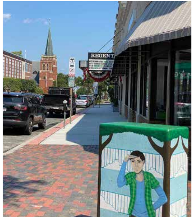
New sidewalks framed with faux brick improve accessibility while giving a nod to historical elements are a feature of the Arlington Center Sidewalk Project
