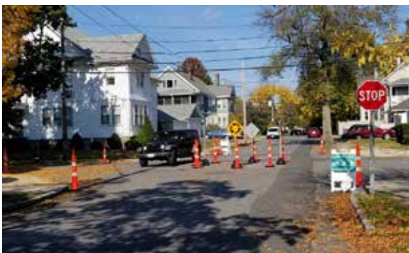
Temporary roundabout piloted at intersection of Mary Street and Burch Street - photo Phil Goff
