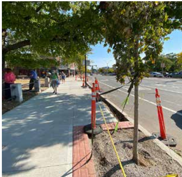
New sidewalks in Arlington Center were installed over the summer.
