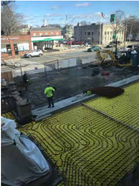
Sub-slab snow melt system being installed at Town Hall Plaza
