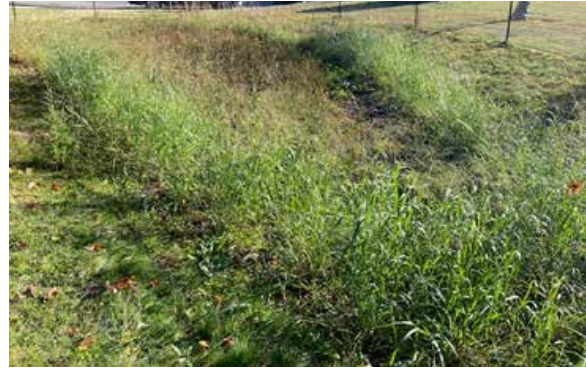
The Spy Pond Project included constructing a biobasin next to Scannell Field to improve stormwater quality before entering Spy Pond.
