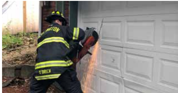
Garage door forcible entry in progress.
