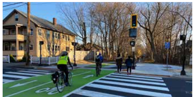
New traffic signal at Lake Street and Minuteman Bikeway.
