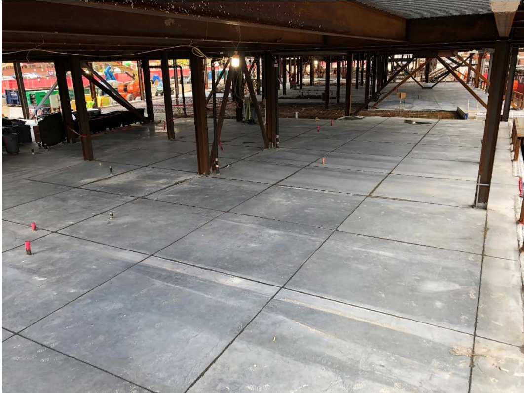
Photograph 3: Building D Slab on Grade
