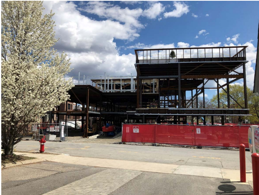
Photograph 2: Phase 1 Progress Photo from Schouler Ct.
