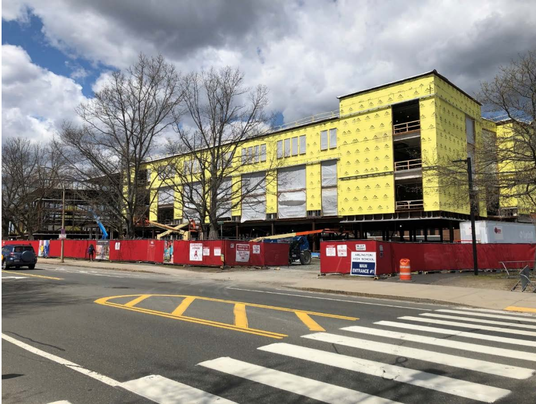
Photograph 1: Phase 1 Progress Photo from Mass Ave
