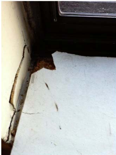
Water damage at jambs and sills at interiors of two apartments
