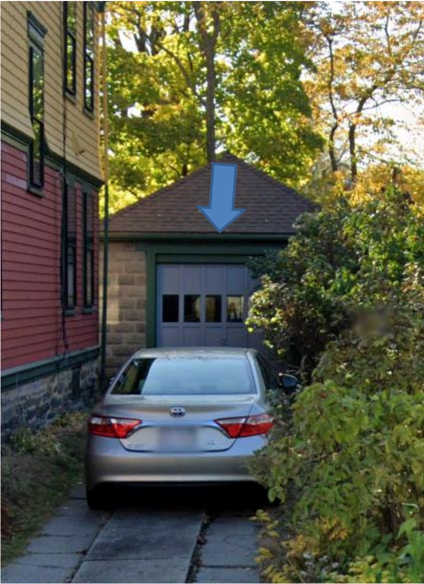
Figure 1: Location of door on garage to be replaced with wood door per attached specs.
