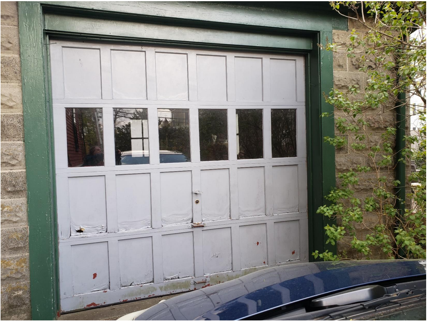
Figure 4: View of Existing Garage Door
