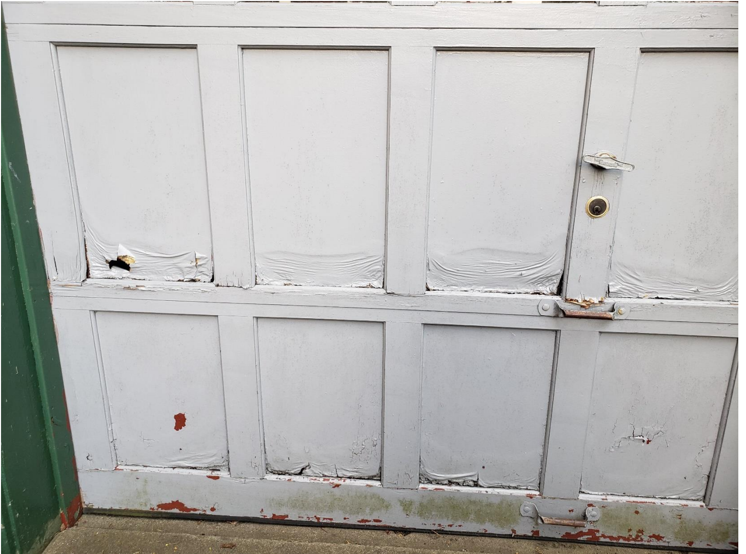
Figure 5: Condition of Existing Garage Door
