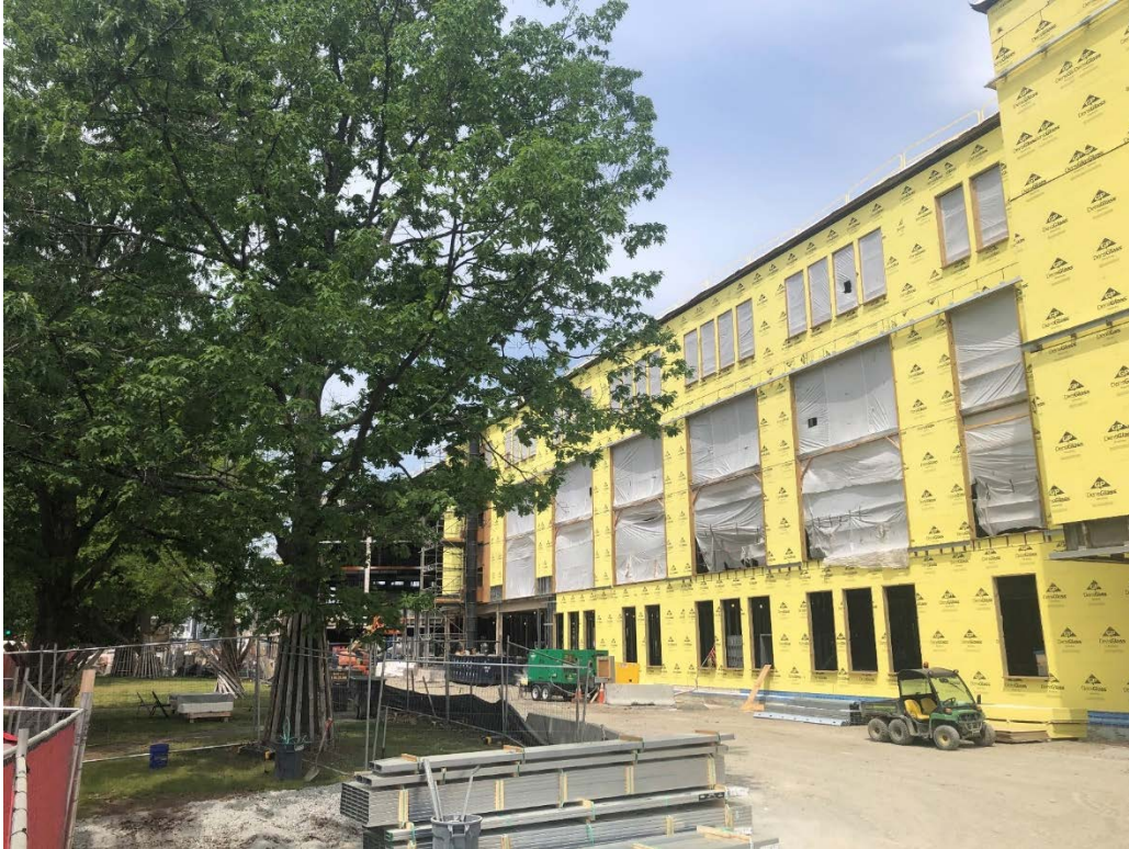
Photograph 1: Phase 1 Progress Photo from Mass Ave
