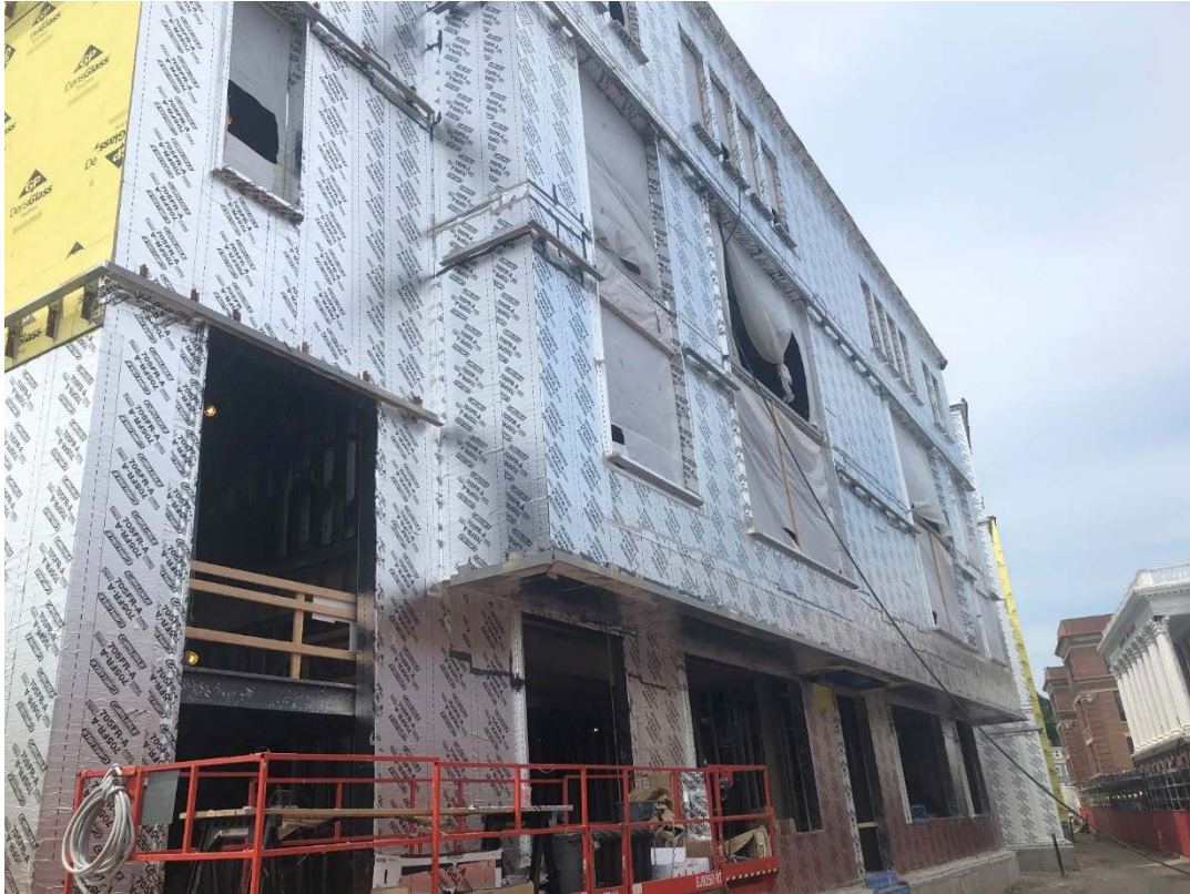
Photograph 5: Air Vapor Barrier (AVB) Progress North of Building D
