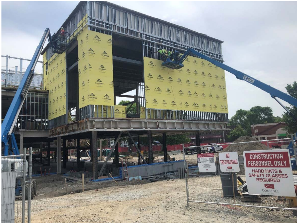
Photograph 2: Phase 1 Progress Photo from Schouler Ct.
