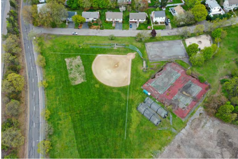
Removal of Poets Corner Tennis Courts
