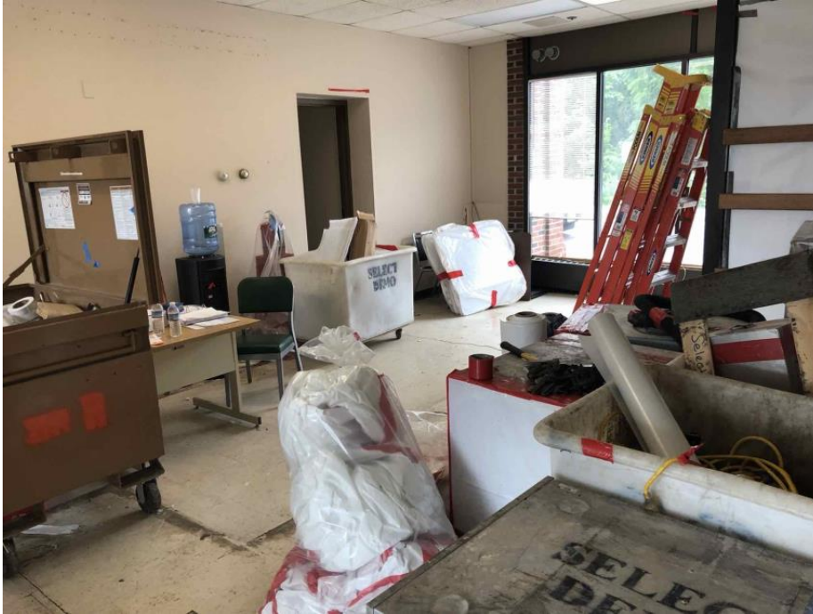
Phase 1 – Demolition at Building A
