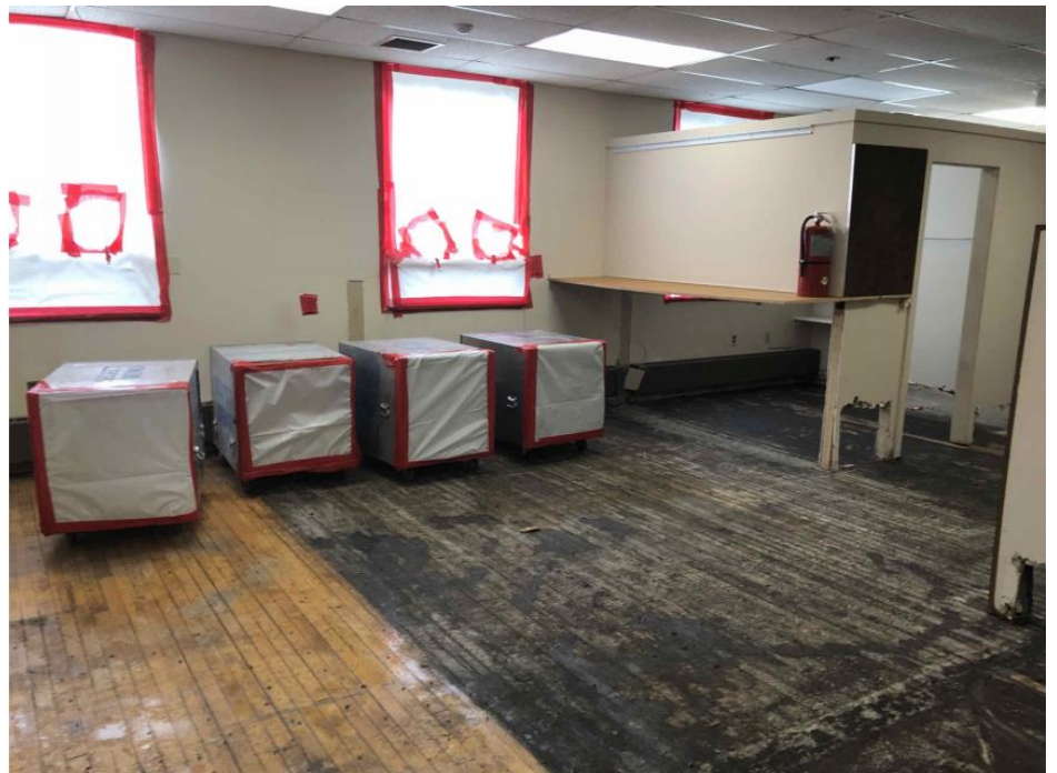
Phase 1 – Demolition at Building A
