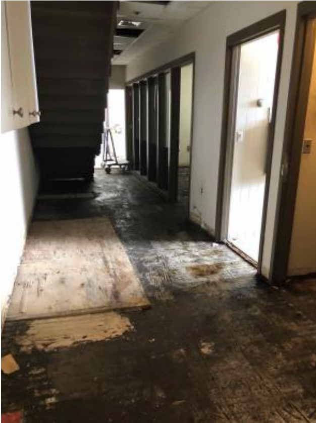
Phase 1 – Demolition at Building A
