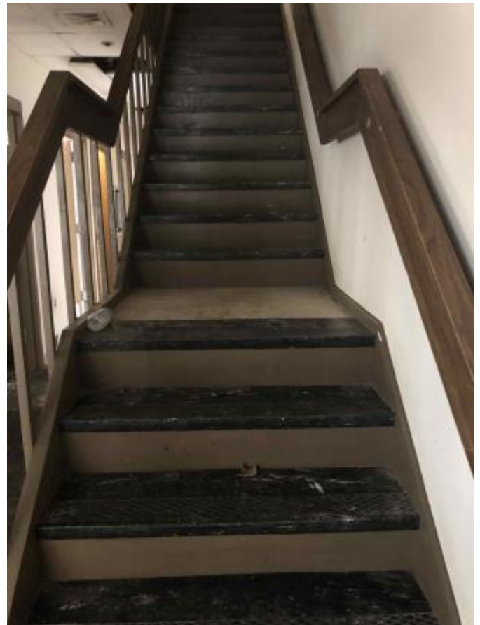
Phase 1 – Demolition at Building A
