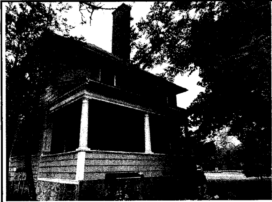
Flat Roof front and right-side porch Sample #20 A, B, C
