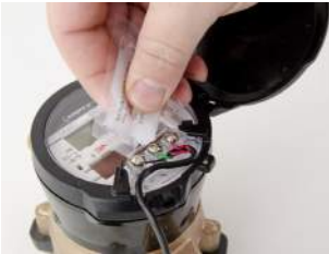
Figure 5 Applying Compound
